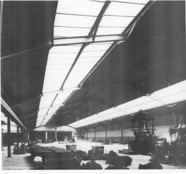
This steel portal roof, which was designed on the plastic theory, is interesting for its lightness (bays are 66 ft. by 25 ft.) but also for the fact that it was the subject of careful cost comparisons against alternative designs and showed a saving of 3s. 4d. per sq. ft. (i.e. a total saving of  $\pounds$ 7,000) over its nearest rival.
