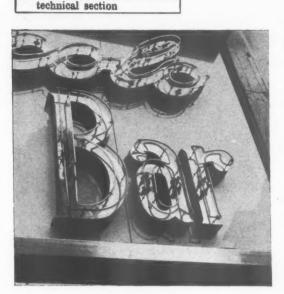
Fig. 4. Double outline tubing superimposed on built-up letters.
