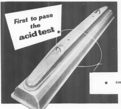
This outstanding development in lighting equipment by the manufacturers of the worldrenowned THORLUX range of lighting fittings will be specially welcome to those industries suffering from the effect of chemically laden atmosphere on metal parts. The new Fibreglass 'Thorlux Acidproof Reflector', for one or two 80-watt fluorescent tubes, is completely resistant to acids met with in the industries listed. Write for specification and prices.
