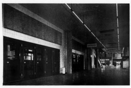
From the concourse passengers walk down this broad corridor to pass through the immigration hall if on a customs flight, straight out to the pier if not. The floor is of dark green terrazzo, the wall finished with 8-in. × 5-in. light grey Belgian semi-glazed tiles, and the ceiling of perforated asbestos-based tiles. The doors to the telephone booths are of dark natural mahogany and of a standard of joinery one had considered lost for ever. The ply panels over are mounted proud of the tiled
