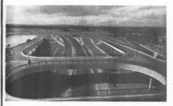
The decision to place the buildings over the junction of the communications entailed the construction of a raised concrete roadway with ramps up from both lanes of the new dual carriageway main Brighton road. Construction is normal reinforced concrete with ramp columns at 40-ft. centres and 16-ft. apart carrying roadway 24-ft. wide.
