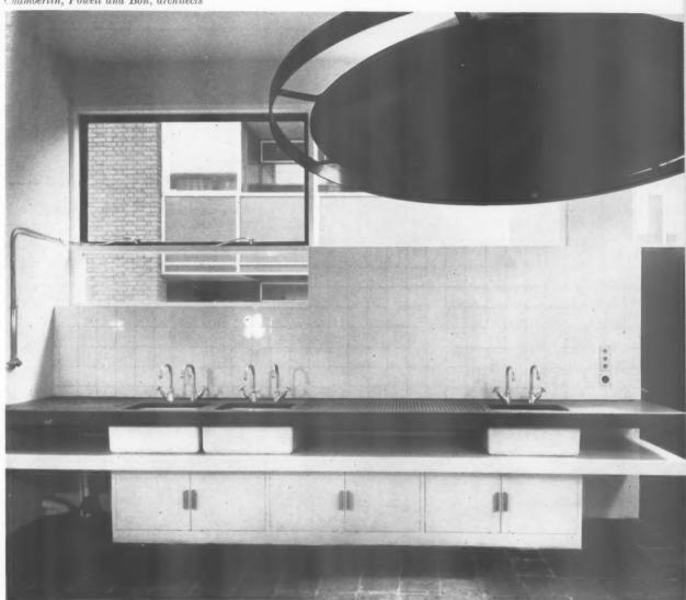
The grooves in the draining boards fall towards the back of the unit where they drain into a channel which has one outlet connected to the waste of one of the sinks.
