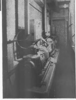
Three of the seven 21 kW motor generator sets associated with each lift installation,
