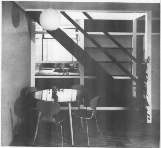
This simple open staircase has  $\frac{1}{2}$  in. dia. m.s. tie rods between treads. The heads of these rods and of the screws which fix the treads are sunk and pelleted.
