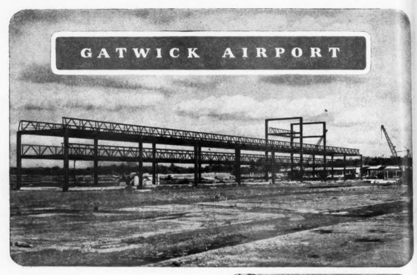
Hotchkiss Lattice Girders of welded tubular construction were supplied for the Central Pier.
