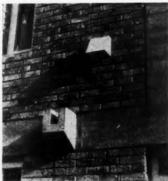
Brick and Concrete at Ham; a detail of wall, floor-slab, ventilator and gargoyle from a new flat development at Ham Common by James Stirling and James Gowan.
