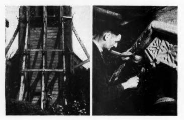
Above left, firm shoring and continuous support by means of close boarding used to support bulging flint walling. Rede church tower, Suffolk. (Architect, Marshall Sisson) Above right, Westminster Abbey. The cleaning of interior stonework with pumice dust and a very limited amount of water—to avoid damage to furniture and fittings. (Architect, S. E. Dykes Bower).
