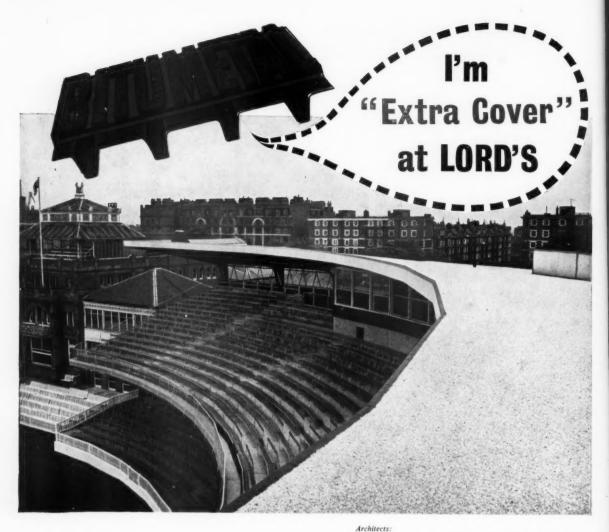
When the Warner Stand was built at Lord's Cricket Ground it was roofed with "BITUMETAL." "BITUMETAL" Aluminium Roof Deck ensures light clean construction, complete freedom from maintenance and a bright ceiling of attractive modern design. It also provides efficient insulation, and a durable weatherproof surface which can be laid in a range of natural colours.
