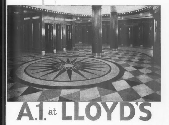
THE RUNNYMEDE RUBBER CO. LTD. are proud to have supplied all the rubber flooring in the new Lloyd's building in Lime Street. A special gauge of rubber,  $\frac{1}{2}''$  thick, was produced for this purpose.
