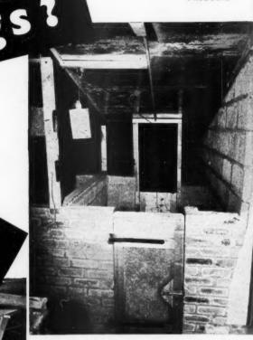
"Paramount" Insulating Plasterboard employed to line roof of a piggery.
