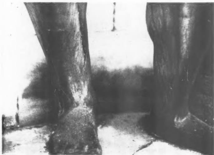
Lead statue burst by rusting of the iron armature (Kedleston Hall, Derbyshire). The only remedy is renewal of defective portions of the armature, taking special precautions to avoid future moisture penetration.
