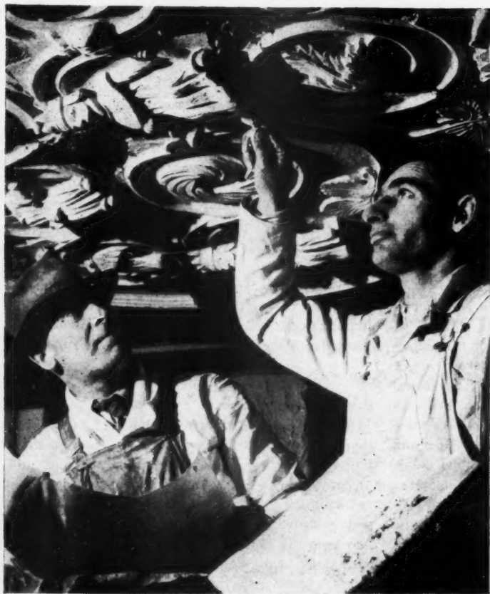
Left, re-fixing a Jesse ceiling on metal lath. (Both photographs on this page supplied by MOW.)
