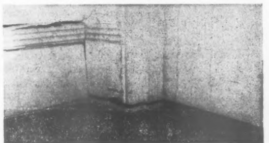
Below, the dropping of floors is frequently caused by dry rot in wall plates and may be detected by cracks at skirtings.
