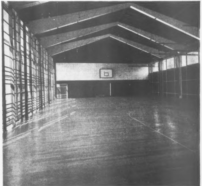
'WOODWELD' PORTAL FRAMES supplied for the Quarrendon School, Aylesbury. Roof Span 47' 6" Consultant: Mr. D. W. Cooper, B.Sc., A.M.I. Struct. E.
