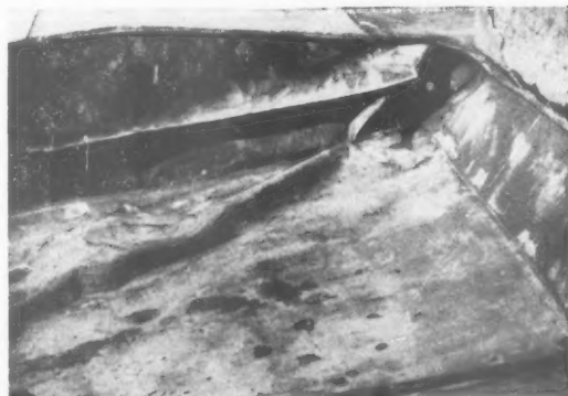
Below, buckled copper roofing (Wotton House, Bucks.) caused by excessive sheet sizes.
