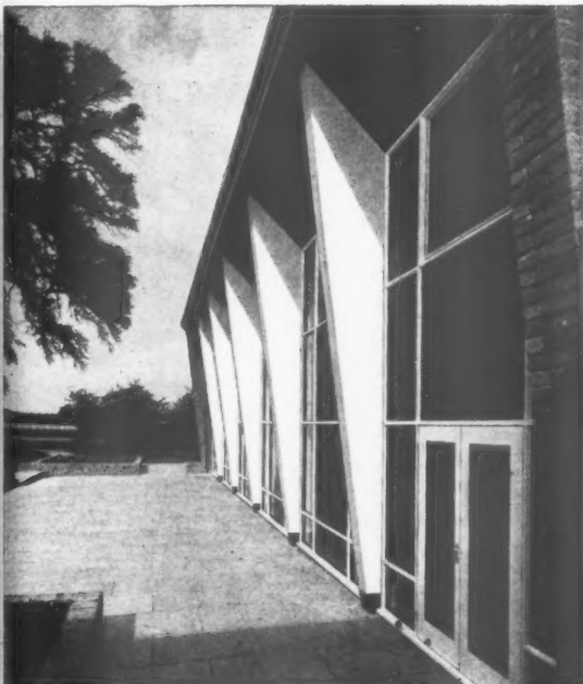
'WOODWELD' PORTAL FRAMES supplied for the Quarrendon School, Aylesbury. Roof Span 47' 6" Consultant: Mr. D. W. Cooper, B.Sc., A.M.I. Struct. E.
