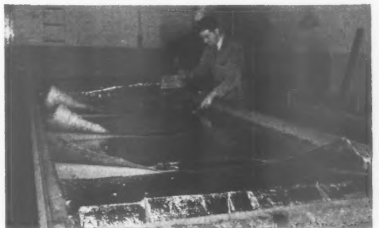
The recasting of sheet lead. Above, a cascade of molten lead is poured on the casting table. Below, lead on the casting table which has cooled and is being cut up into suitably sized pieces. Bottom, lead burning. (Lower photographs by courtesy of MOW).
