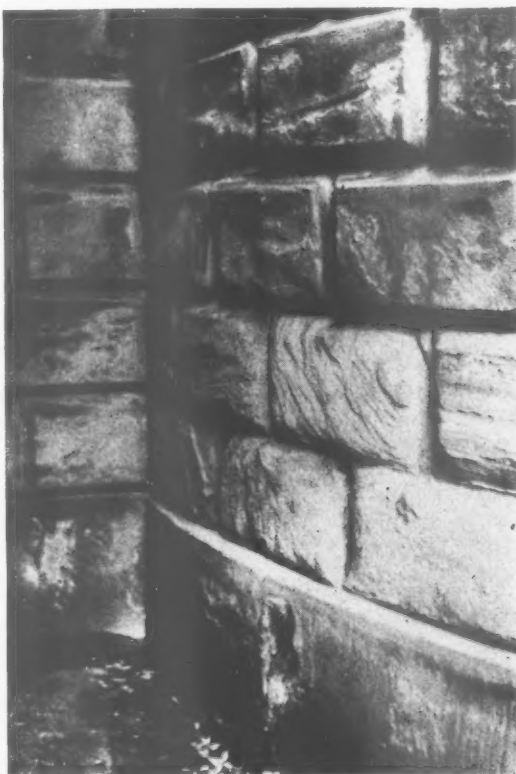
Above damage to soft sandstone by mason bees. Below, wind erosion of stonework caused by eddies in a re-entrant angle.
