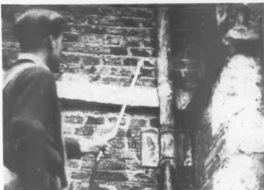
Sterilising brickwork affected by dry rot. Holes have been drilled into the joints, and the brickwork is heated and then saturated with fungicide.
