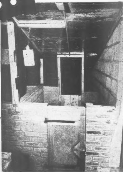
'Paramount' Insulating Plasterboard employed to line roof of a piggery.
