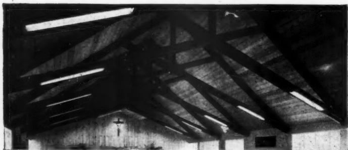
Fig. 18. Interior of Church at Agassiz, BC, by Gardiner and Thornton, showing scissor truss.
