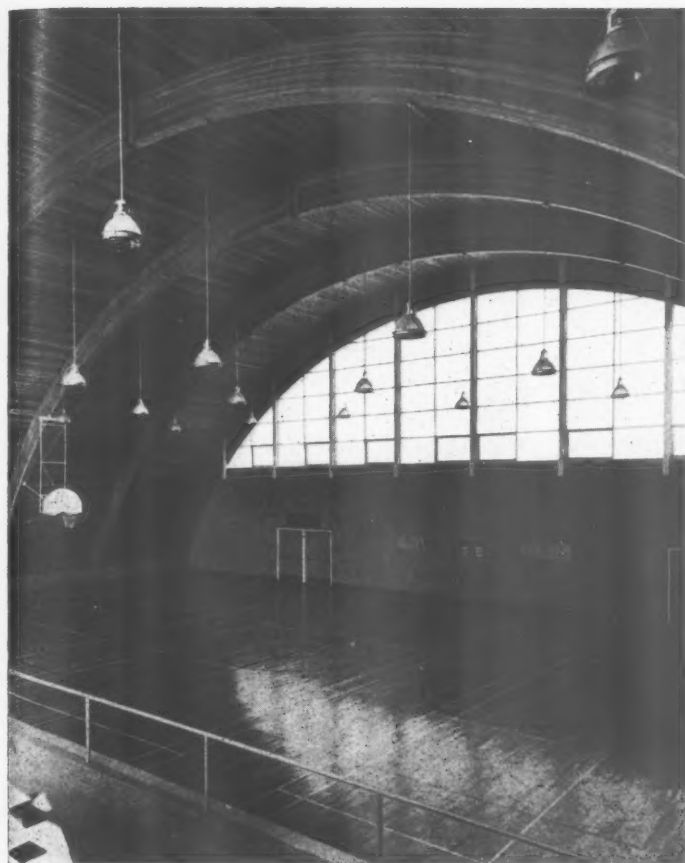
Fig. 20. Glued laminated arches in the University Hill School gymnasium by Thompson, Berwick and Pratt.
