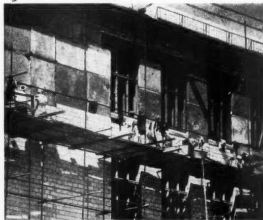
Fig. 16. Women building workers tiling the exterior of the Kiev school. The load-bearing external walls are built of large crane-handled slag-concrete slabs.
