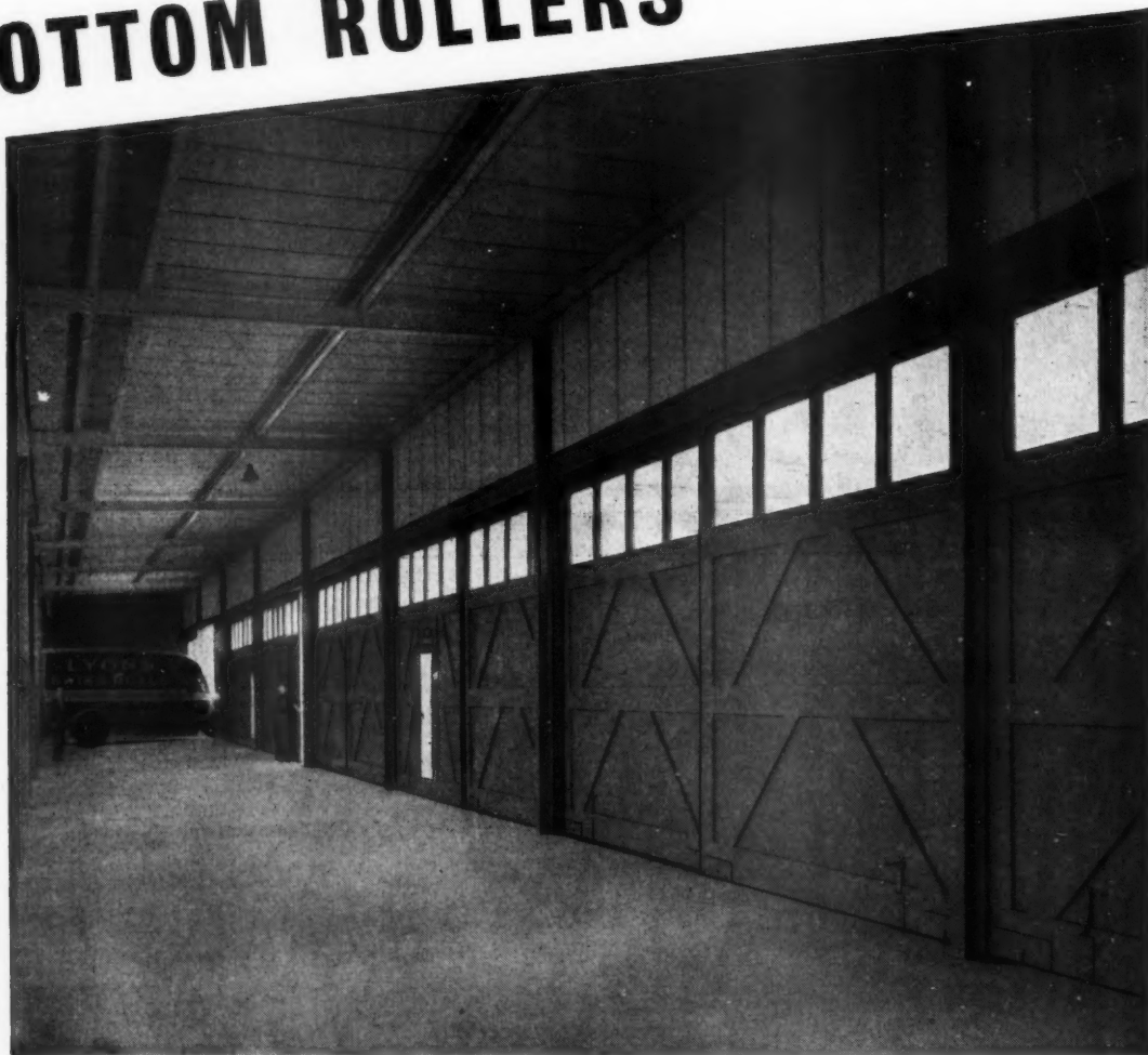
Double line of passing doors in a despatch building.
