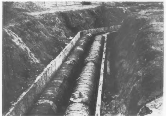
Fig. 65. More than 160 Russian towns now have district heating schemes. This photograph shows insulated district heating mains, about 2ft. 6 in. in diameter, being laid in a suburb of Moscow. The duct is subsequently covered with precast concrete units.
