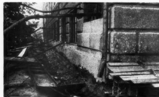
Fig. 21. Temporary flexible connections passing through the basement windows enable all services—gas, electricity, sanitary plumbing, water, heating, telephones—to be maintained during the moving of the building.
