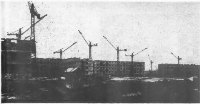
Fig. 53. A massive array of tower cranes at Chokolivka, where the organization of building was said to be on the "continuous flow" method (see text). Behind the spoil heap in the foreground, in surprising contrast to the mechanization going on in the background, were a group of about twenty women carrying out excavation by hand.
