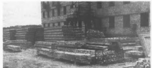
Fig. 56. Hollow precast floor slabs stacked ready for crane-hoisting.
