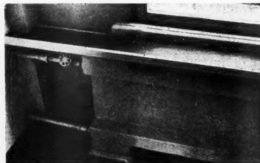
Fig. 37. A reinforced concrete radiator under a kitchen window sill. See Fig. 29 (7).
