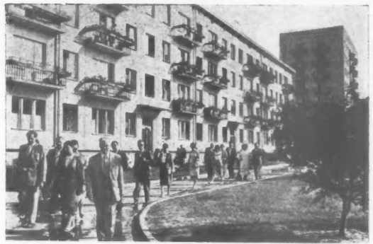
Fig. 30. Blocks Nos. 8 and 13a. The point block walls are cream-painted slag-concrete panels. The lower block also has precast wall panels painted. Undersides only of balconies are painted in primary colours.
