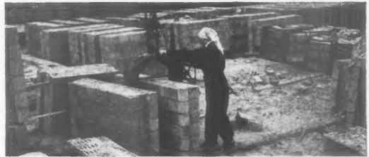
Fig. 55. A girl worker preparing a brick walling-slab for hoisting by a tower crane. Owing to the multiplicity of different kinds of wall panels, it sometimes takes quite a long time to find the right one—an acknowledged disadvantage of the system.
