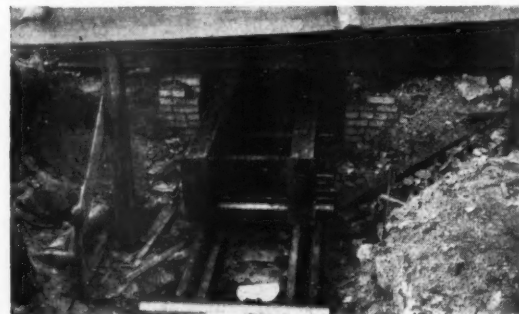
Fig. 20. Steel rollers being placed under the r.s.j. framework on a track along which the building will be pulled when it is ready to be moved.
