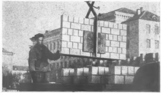
Fig. 54. A lorry load of factory-made brick walling-slabs.
