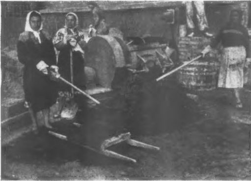
Fig. 22. Women building workers on a housing site at Kiev. The tool in the foreground is a hand-carrier, or barrow without a wheel, for carrying by two workers. It is surprising to see such equipment on a site which, at the same time, is heavily stocked with tower cranes, and prefabricated wall components.
