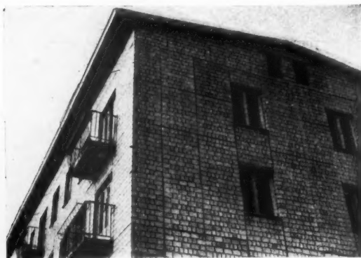
Fig. 36. Detail showing factory-made brick wall "slabbing."
