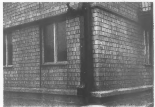
Fig. 57. Detail on the ground level of a block of flats built of factory-made brick slabs. The enormous rainwater pipe is said to be to cope with snow and ice. Now that in the latest blocks plumbing is being cast in to wall panels, arguments have been found for reducing the pipes in size.
