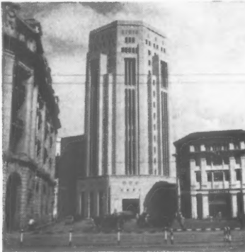
BANK OF CHINA SINGAPORE Architects: Palmer & Turner
