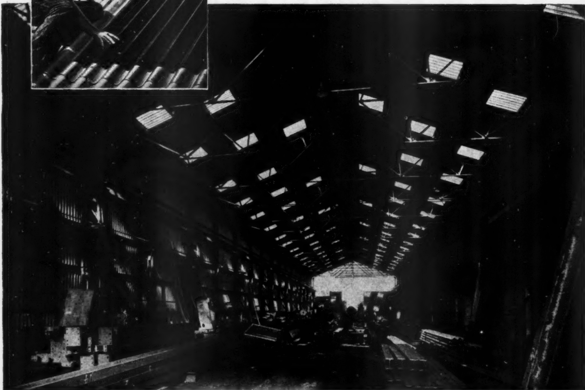
An interior view of the Corrugated 'Perspex' installed over 8 years ago at the works of Henry Smith (Constructional Engineers) Ltd., of Winsford, Cheshire.
