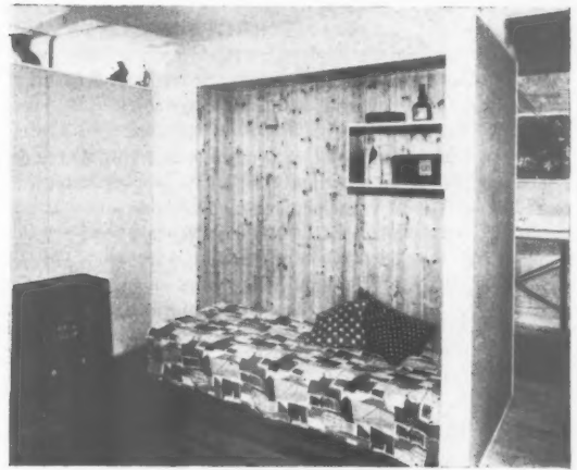
A corner of the living room of the house at Stanway Green. The general wall and ceiling finish is of fibreboard painted with emulsion paint; the recess is lined with softwood boarding. Some external walls are left with wood wool exposed internally. The floor is of softwood boarding.
