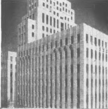
OFFICES FOR TRANSVAAL & CHAMBER OF MINES JOHANNESBURG Architects: K. E. F. Gardiner & MacFabgden
