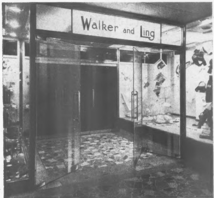
Entrance doors with sidelights at Weston-super-Mare. Special spring and hinge unit with retractable pivot allows door and sidelight to be folded back.
