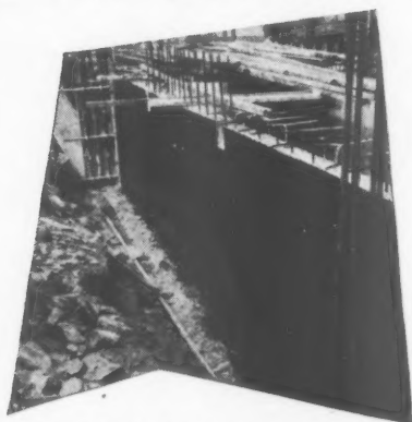
A typical basement tanking.
