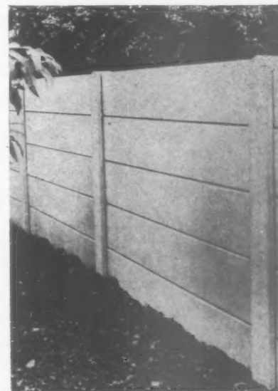
Below, Marley post and panel concrete walling.
