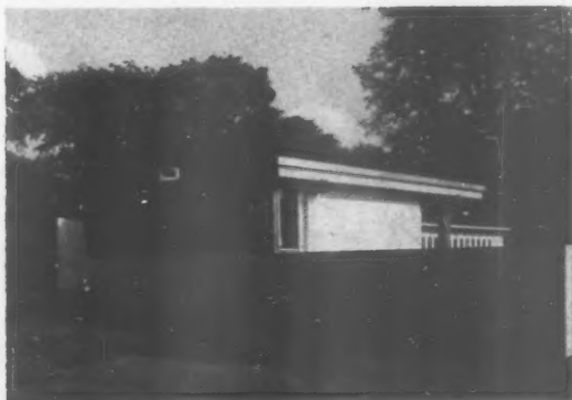
Below left, the north-west corner of the house. The large window at the far end is to the living room; a low stone retaining wall forms a small terrace here. The continuous run of windows is to the kitchen, bathroom and bedroom. The brick wall underneath is carried out as a screen wall, and takes up a slight difference in ground levels.
