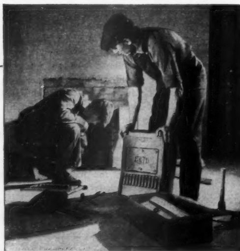
Bacboilers like this are being installed in new homes at Aycliffe.
