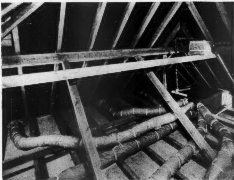
Potterton warm air unit showing ducts: ceiling not insulated.
