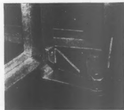
Crittall's galvanized window fitted with a friction hinge.
