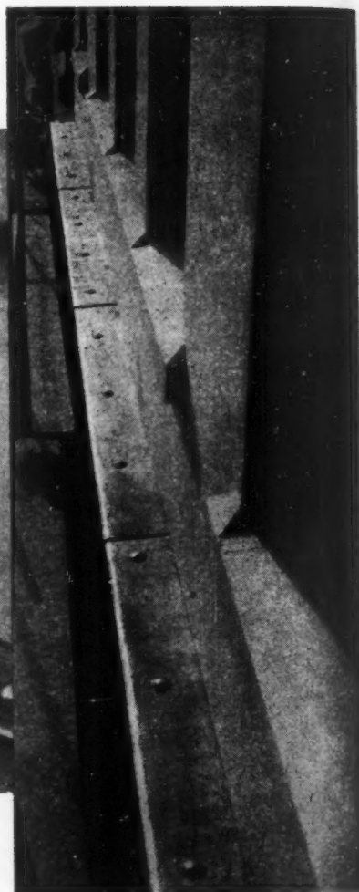
A typical example of lead weatherings for stone-faced buildings. New office building, London W.1 Architect: H. G. Sumner, L.R.I.B.A.
