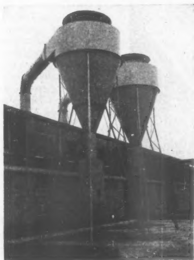
Cyclone separators for foundry fettling benches
