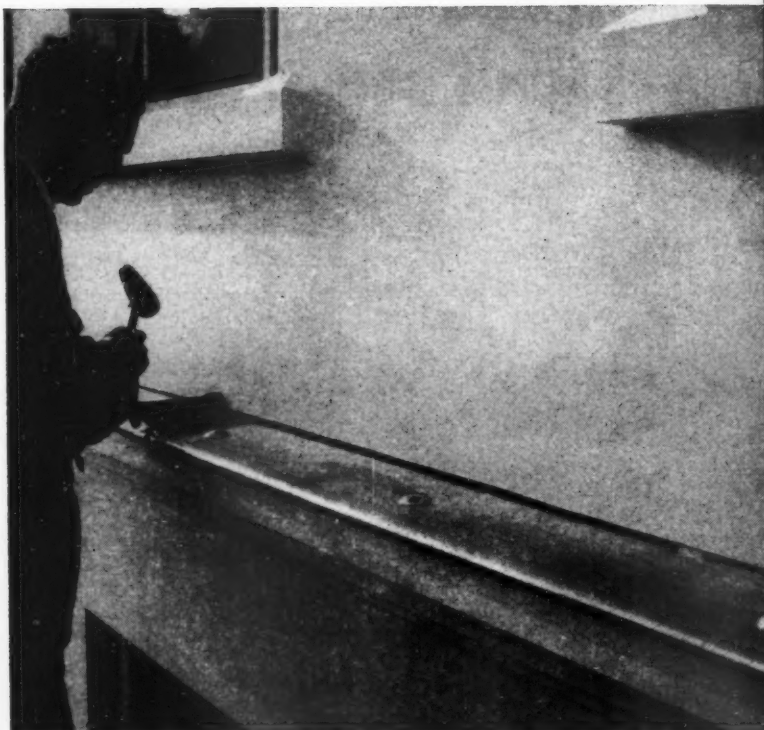
A typical example of lead weatherings for stone-faced buildings. New office building, London W.1 Architect: H. G. Sumner, L.R.I.B.A.
