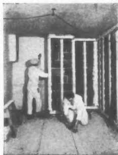
Paramount Plasterboard used as a lining to traditional walls.
