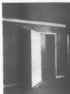
Paramount Cove used to mask junction of walls and ceilings in a modern bungalow. No unsightly cracks.
