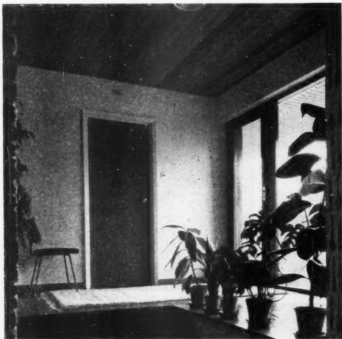
The entrance hall from viewpoint 4. The ceiling, like the eaves soffits, is of tongued and grooved softwood boarding.
