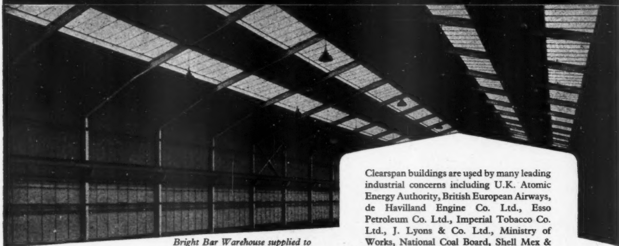
Bright Bar Warehouse supplied to Arthur Lee & Son Ltd., Sheffield. Length 225 ft. Span 80 ft. 5 ton crane
