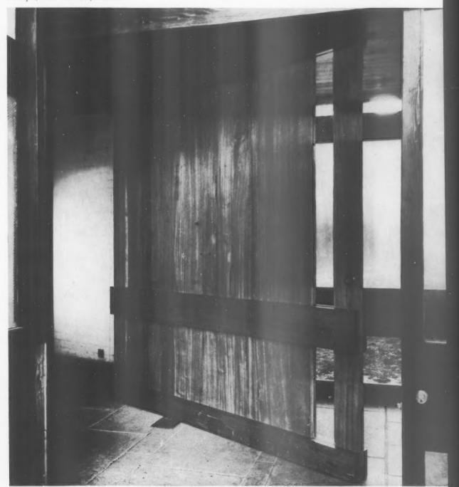
This pivoted door is fitted with a double-action door spring to hold it open at 90°. There are no door stops as the floor spring and the weight of the door are sufficient to hold it stationary when open. The wood is British Columbian pine. The centre rail provides a hand-pull on the inside where it crosses the vertical strip of glazing and the corresponding "blind" recess at the other end of the door.
