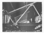
2. Paramount Insulating Plasterboard employed as a fire-safe roof lining in a new factory. They make matches in this one.
