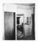
1. This photograph shows Paramount Plasterboard used for dry lining of external walls ready to receive the finished decoration. It also shows the use of Paramount Dry Partition consisting of 2 sheets of Paramount Plasterboard separated by a cellular core to which they are inseparably bonded. The use of Paramount Plasterboard for the ceiling will be noticed, and also of Paramount Cove, a section of which is lying, in the bottom left-hand corner.
