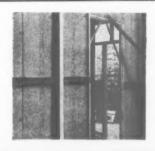
6. Paramount ‡" Plasterboard for 2" solid partition, being erected as a fire stop in a large undivided factory.
