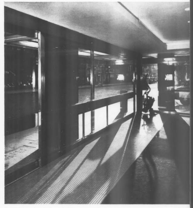
The framing of these magnificent sliding doors is built up from a pressed steel core, made out with sections of hardwood and clad with stainless steel. Both the beads and the pelmet boards which conceal the overhead gear are likewise of hardwood clad with stainless steel. The doors slide back into  $\pi$  void and when fully open leave an unobstructed opening (unobstructed, that is, except for the freestanding column) of over 33 feet.
