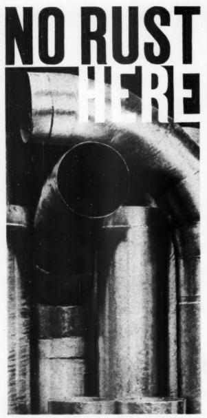
These ducts are safe from rust because they are hot galvanized, the most effective method of preventing the corrosion of iron and steel and the cheapest in the end. Hot galvanizing ensures a tough, tightly adherent & thick coating of zinc alloyed to the basic steel. Few structures or parts are too big, too small or too complex for this versatile process. For further information write to the Hot Dip Galvanizers Association, 34 Berkeley Square, London W1
