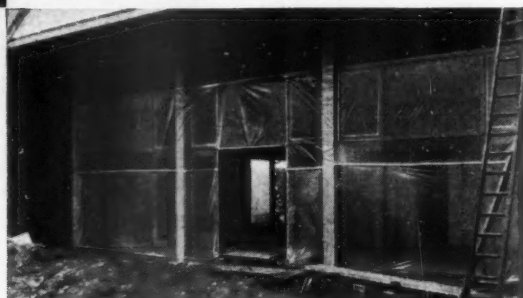
Gilbert Ash Ltd. used 'Visqueen' during the construction of a new canteen at the English Electric factory in Stevenage. Temporary glazing enabled plastering, electrical fittings and wooden flooring to be completed on schedule unaffected by bad weather and without risk of damaging specially fabricated expensive plate glass.
