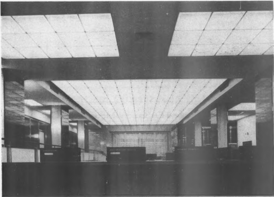
The main working area of the bank. 231 two-foot square Lumenated Module panels are used for the lighting installation.
