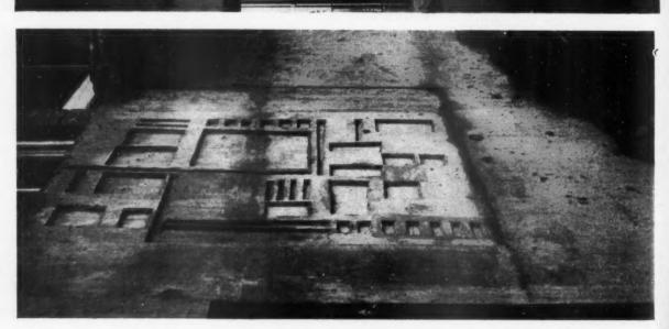
William Mitchell in their decorative work done in collaboration with the LCC's housing architects are shown here: extreme left, an example of three dimensional patterning in poured concrete, obtained by applying wooden forms to the shuttering, used on the ground floor walls of two eleven-storey flat blocks at Derby Hill estate, Lewisham. Left, painted cement shapes made by masking
