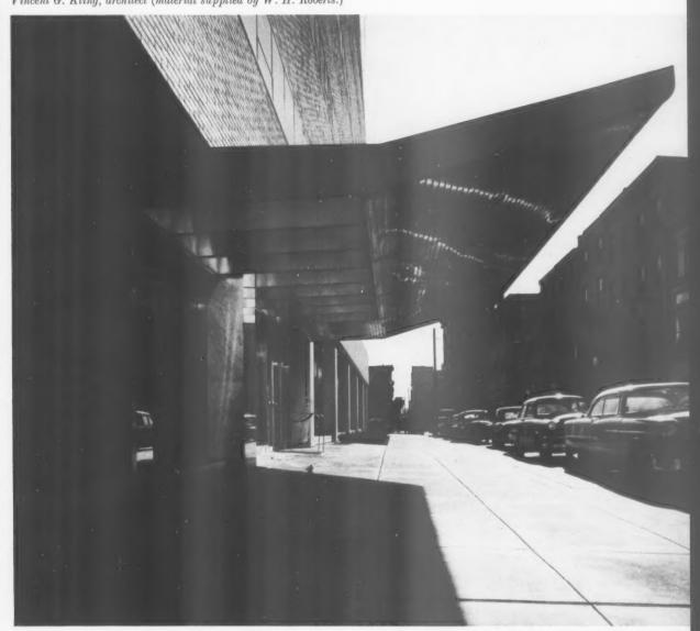
This deep canopy, with open light well at the wall face, has a form reminiscent of timber, but is in fact of stainless steel, the main rafters being formed of box beams 1 ft. 6 in. deep and 3 in. wide.
