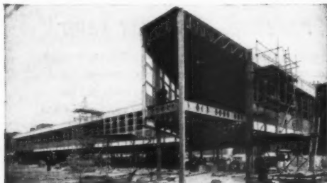
New Air Terminus buildings in Kensington for B.E.A. Photograph taken 16 days after commencement of steel deliveries. Main Contractors: Messrs Richard Costain Limited.
