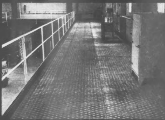
A complete gallery fabricated in rectangular punched Alaflor and installed in a new extension to the Radio Chemical Laboratory, Teddington, Middlesex.
