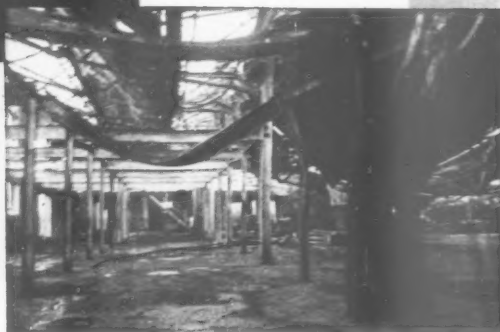
BELOW: Distortion by fire of unprotected steel beams and columns.
