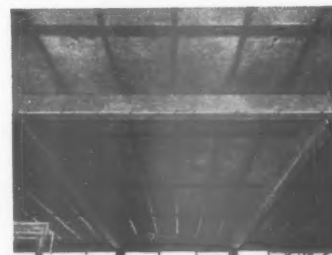
10. Steel columns and beams protected with Paramount Plasterboard and fixed with Blue Hawk R.S.J. Clips in a garage at Coventry. Erected AFTER the Jaguar fire.
