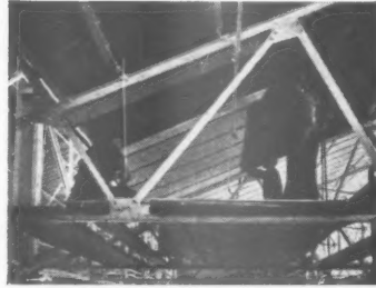
2. Paramount Insulating Plasterboard employed as a fire-safe roof lining in a new factory. They make matches in this one.
