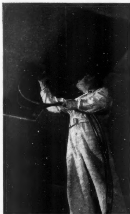
Tretoplast coating being spray-applied to a prepared area of ceiling
