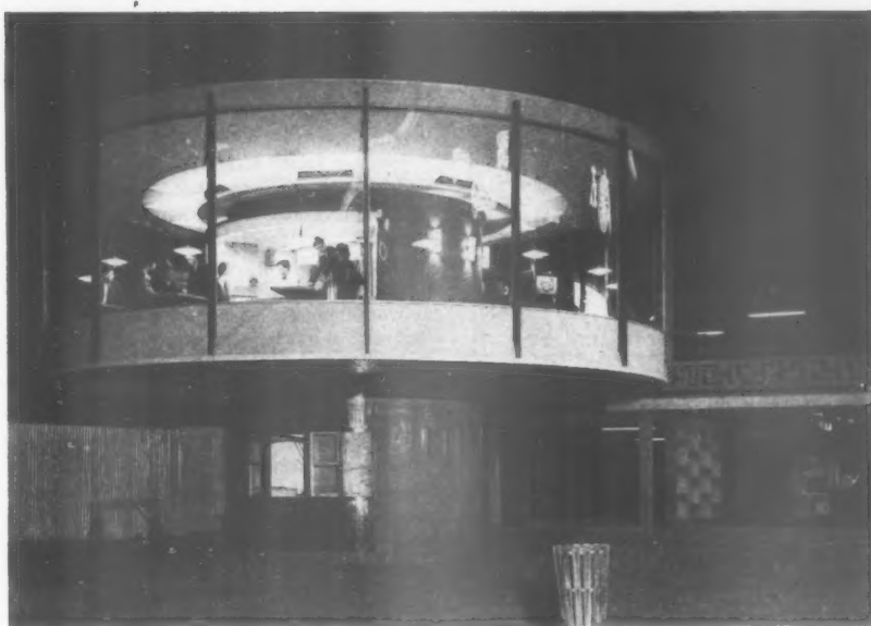
The circular café in Coventry's pedestrian shopping area. It has concrete walls 6 in. thick. Fascia, spandrel and part of the drum are faced with mosaic. The soffit of the cantilever is of plywood panels. See note, "Can You Get a Square Meal?"
