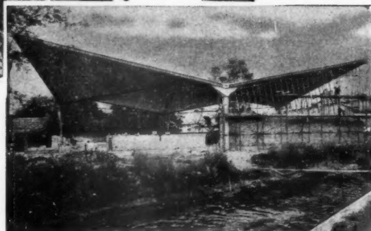
The roof consists of four panels of hyperbolic paraboloid shells, each 57 ft. 5 in. square, supported independently by a concrete column at the mid-point of each side and weatherproofed with Ruberoid Built-Up Roofing.
