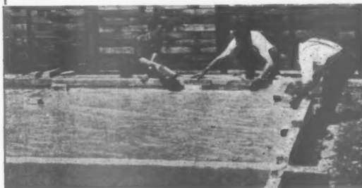
Unity Structures Ltd., London, laying 'Visqueen' 500 (heavy weight) as a damp-proof membrane between the hardcore and concrete flooring of these two semi-detached prototype houses built by them at Ruislip. The film was laid over the hardcore in 12 ft. widths in one continuous strip over the party walls, and incorporated into the cavity wall with the D.P.C.
