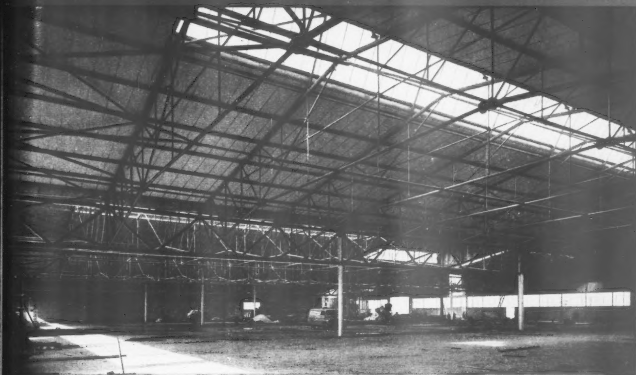
Interior of building showing tubular steel roof structure.
