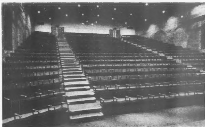
Left: the auditorium seen from the stage. The seats are fixed directly on to the tiered banking.
