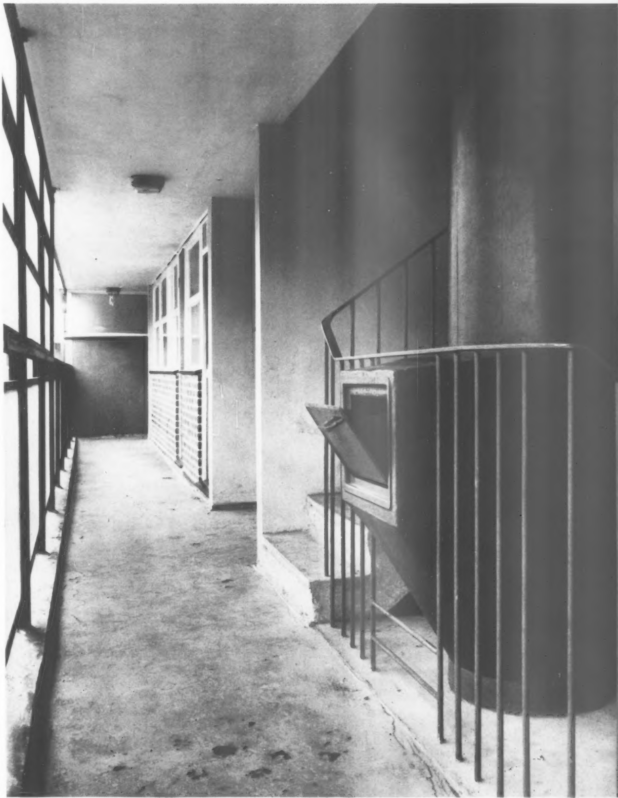
The refuse chute comprises two basic units. The receiving unit at each floor level is precast concrete, purpose-made, into which the standard cast-iron hopper and frame is built. Connecting these units between floors is a standard precast concrete drain-pipe section.
