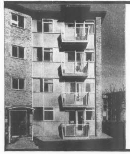
Showing how the balcony floors have been trimmed round the Wallspan mullions.
