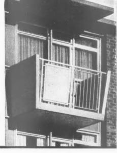
Infilling panels are of ½" Asbestolux faced with stucco-embossed silicon alloy aluminium sheet.
