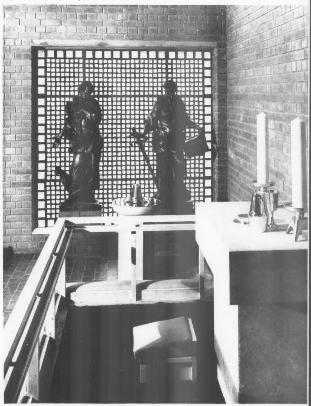
This paraphrase of the traditional stained glass window uses a constructional technique commonly associated with pavement lights. The panes are of strong colours arranged in an abstract pattern.
