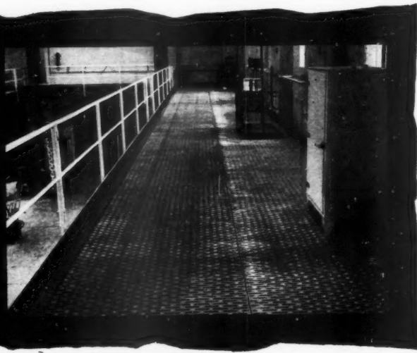
A complete gallery fabricated in rectangular punched Alaflor and installed in a new extension to the Radio Chemical Laboratories, at the National Chemical Laboratory, Teddington, Middlesex.
