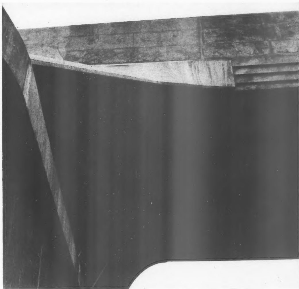
Fig. 15. (Bridge near Ridgmont) . . . a close-up showing the poor concrete finish occurring occasionally.
