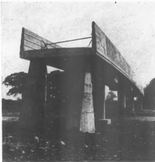
Fig. 19. A bridle road bridge near Ridgmont, with four spans and massive buried supports.
