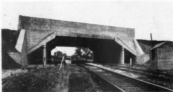
Fig. 17. Precasting has been used in bridges over railway lines where it is essential to reduce the time of occupation of the track. The finish is good but the structural complication for so small a span is grossly exaggerated.
