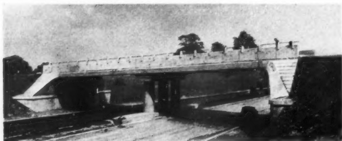
Fig. 14. "If a two span portal in reinforced concrete cast in situ is the right answer, it is difficult to see how it could be constructed more expeditiously."
