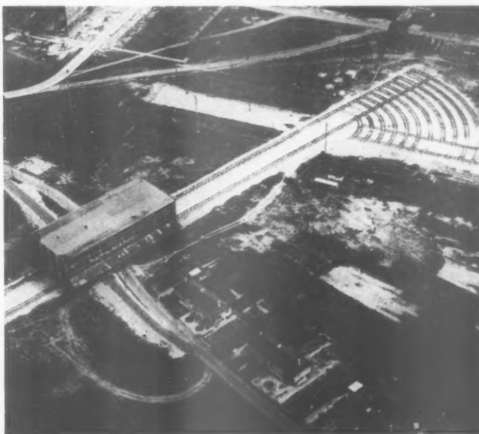
Moving of factory. Note turntable to change orientation.
