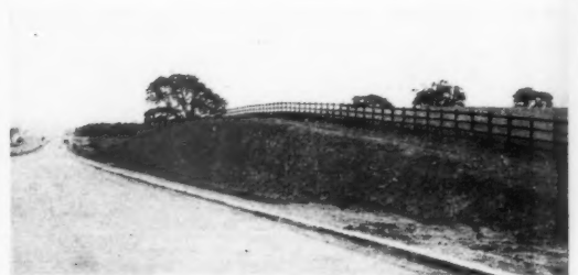
Fig. 4 (left). For reasons of land economy and cost, the banks are graded to an angle of minimum repose, 1:1\frac{1}{2} or 1:2 . This results in an arbitrary wavy line at the top of the cutting. As the ground level view above (Fig. 5) shows, the top of the embankment is emphasized by a fence, later to be reinforced by a hedge. Slight additional shaping would merge the top of the cut with the farmland beyond (view near Eversholt).
