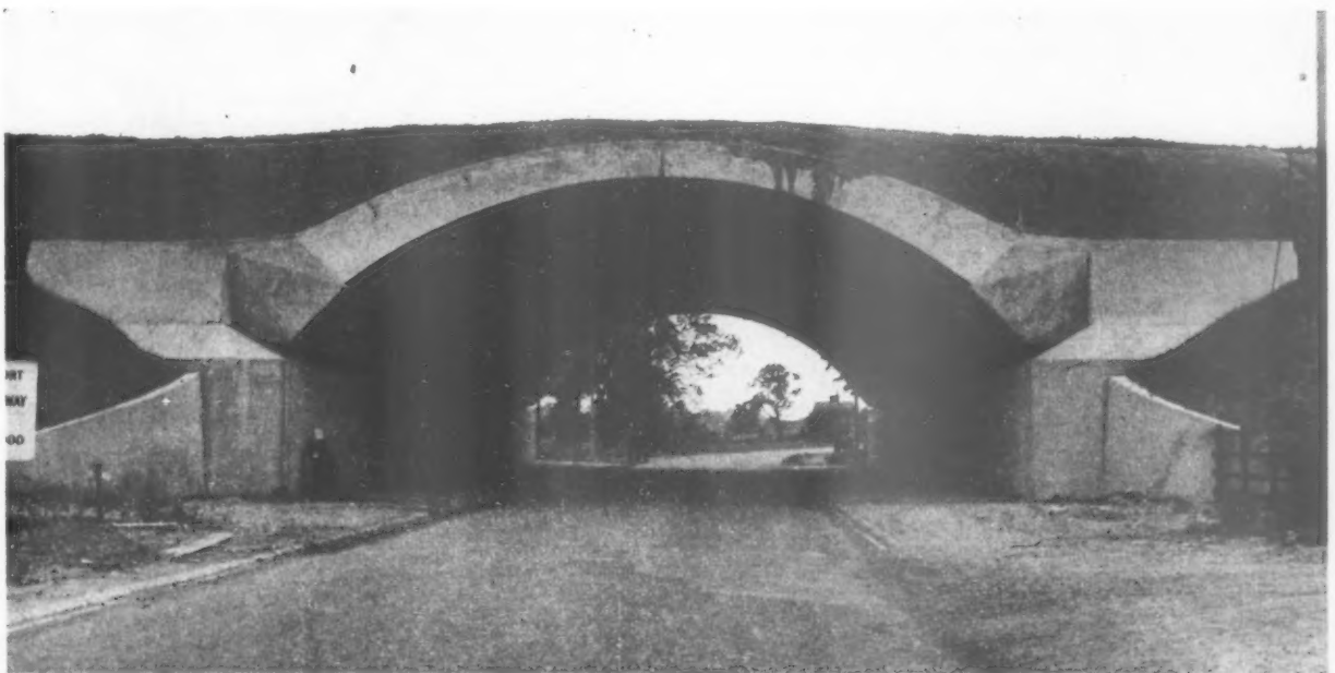
Fig. 20. Some of the bridges are of simple mass concrete and are very impressive. This example is over the Newport Pagnell—Wolveston road.
