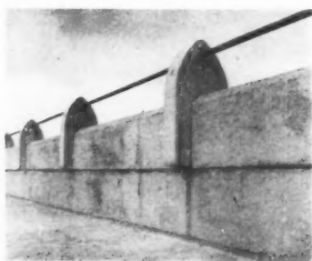
Fig. 13. Where services are carried in ducts under pavements, the parapet walls become too low, so a rail is crudely added.
