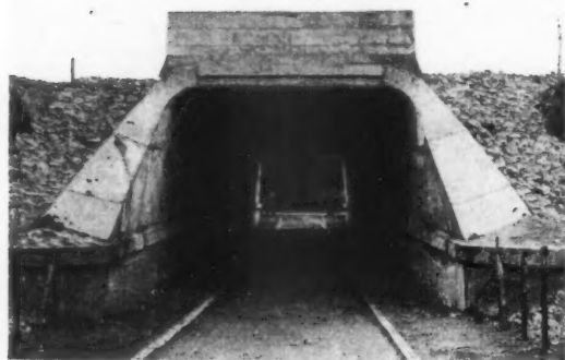
Fig. 8 (above). A square-topped underpass, marked by a solid, ornamented parapet, and with stone-pitching at the sides. Fig. 9 (below). A higher, arched concrete cattle creep, used where head-room permits, which fits in more happily and is not quite so gloomy.
