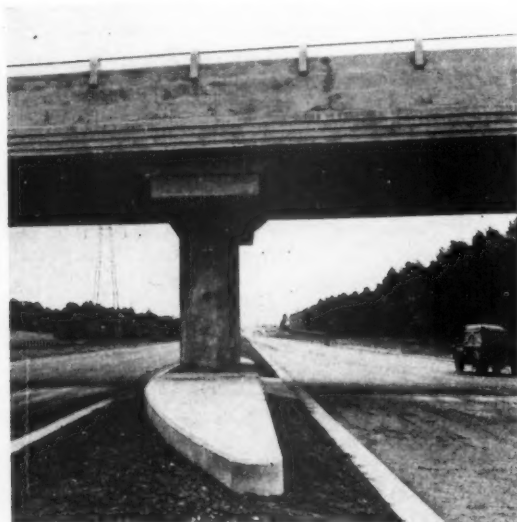
Fig. 18. The standard form of bridge . . . is propped in the middle by gigantic columns. In the foreground is the curving heavy curb to deflect passing vehicles.
