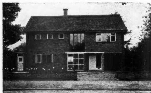
Mr. Brennand's is a cavity-walled house, with double glazing to all windows and doors
