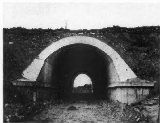
Fig. 8 (above). A square-topped underpass, marked by a solid, ornamented parapet, and with stone-pitching at the sides. Fig. 9 (below). A higher, arched concrete cattle creep, used where head-room permits, which fits in more happily and is not quite so gloomy.
