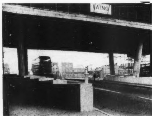
Fig. 11. The offices of the Ringway Centre form a bridge over Hurst Street where it debouches into the Ring Road. Pedestrian subway on left. Note the curious lack of integration between the design of the building and that of the subway and parapets, each being from different offices.
