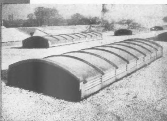
Gable End Continuous Rooflight Ventilators 16 ft. long x 5 ft. 2 ins. wide were installed on the Textile Paper Tube Factory, Romilly, Cheshire. Supplied in extended lengths from 4 ft. with nominal widths up to 7 ft. (Architects: Arthur Swift & Partners.)
