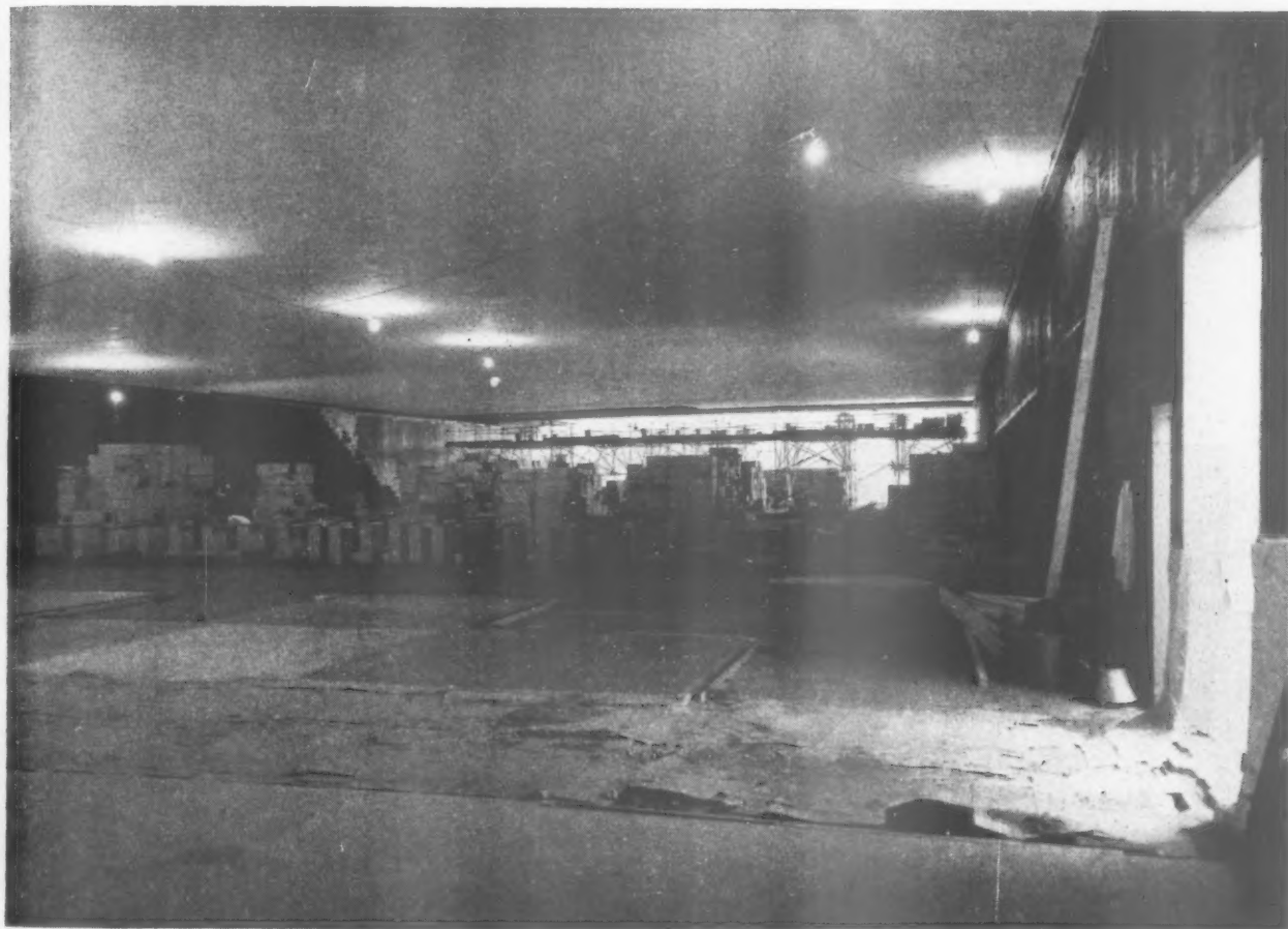
This photograph shows rapid progress on the insulation of a new 580,000 c.ft. cold store for Birds Eye Foods Ltd., at Kirkby Trading Estate, Liverpool.
