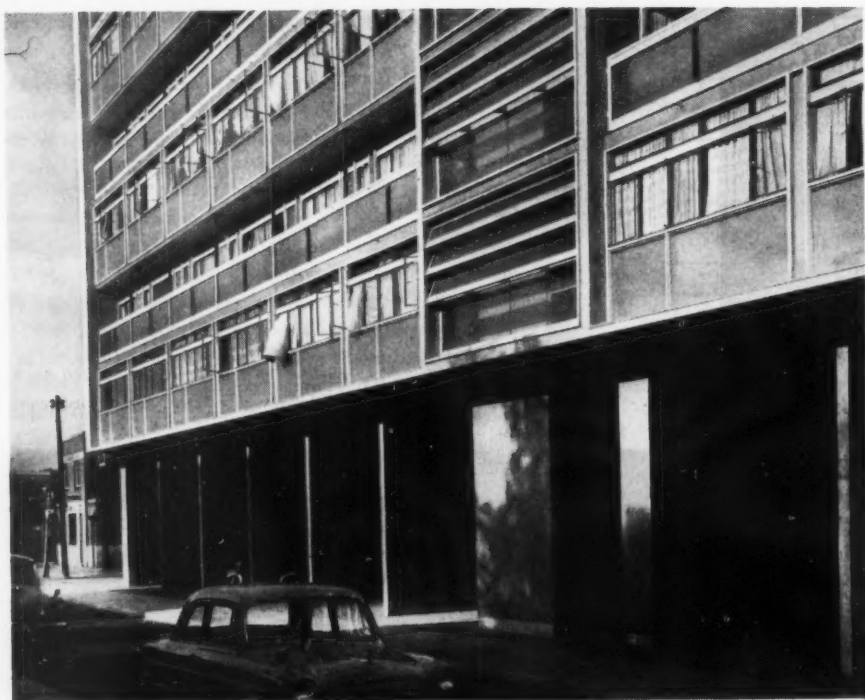
Close-up of service road approach to one of the tall blocks. Note how the crosswalls continuing down through the ground floor hamper the planned use of this area. Below left: the glazed lift shaft of a tall block.
