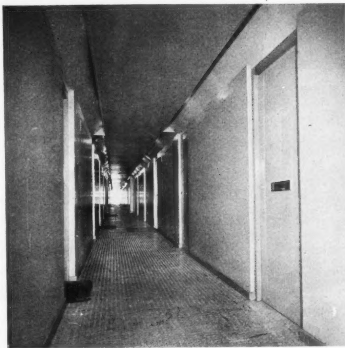
Left: internal corridor in a maisonette block. The first door on right is a front door, the second is an escape door from a bedroom, which does not reach the full height of the recess. Illumination is by a simple system of concealed lighting and the floor is covered with studded rubber tiles.
