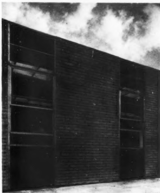
Viewpoint 10 (above): vertical sliding metal windows to control laboratories. Viewpoint 11 (below): tank farm for storage of raw materials.
