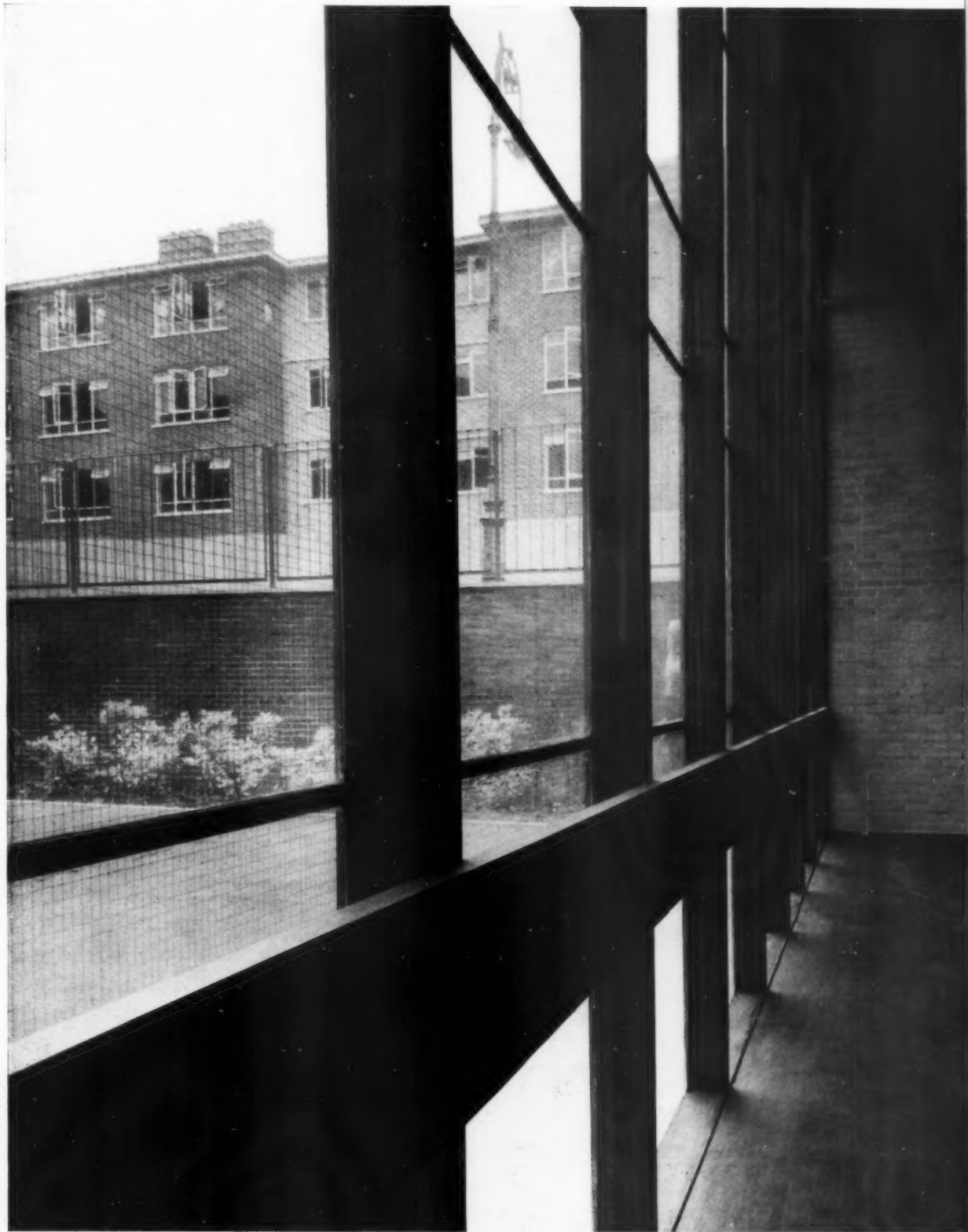
This detail is interesting for its use of timber as an engineering material. Note the laminated timber mullions and beam above. Note also (particularly on the drawing) the exceptionally neat framing to the window.
