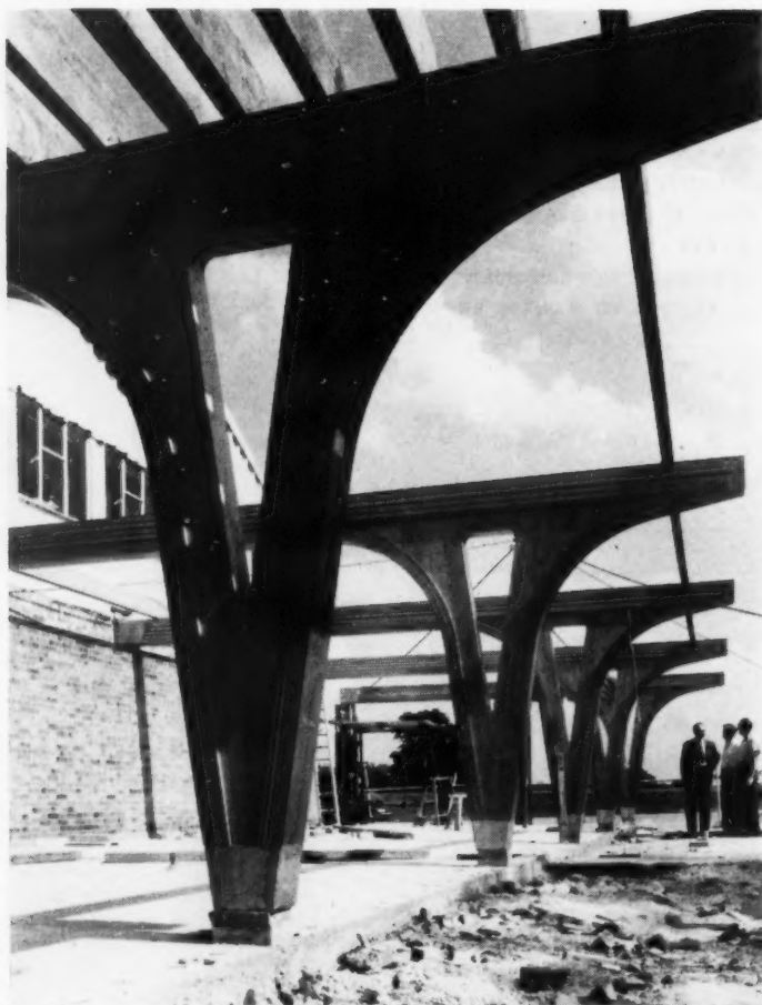
The glued timber Y-shaped columns during building construction.
