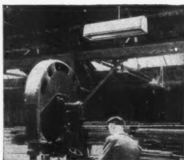
Localised warmth at machines and work benches without the waste involved in heating unoccupied areas, is provided by A.E.I. radiant space heaters.
