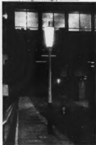
Amenity Lighting Columns with diffuser in .040 'Perspex'. The fitting holds four 2 ft. 40 watt fluorescent lamps.
