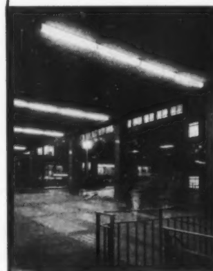
Continuous fittings between columns under low block, with diffuser in .040 'Perspex' with black 'Perspex' ends. Each 5 ft. unit accommodates one 5 ft. 80 watt lamp.
