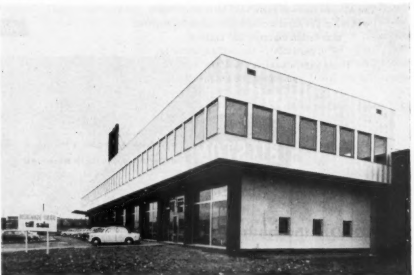
Below, Stenmar aluminium panels on the Fiat building in Stockholm. Above, section showing Vinculum structure unit.
