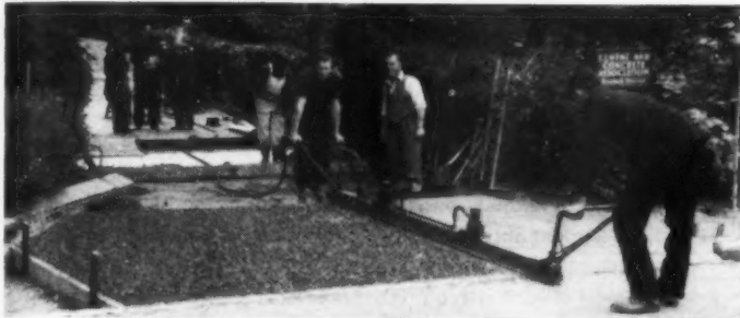
Fig. 2. Pneumatic tamper.
