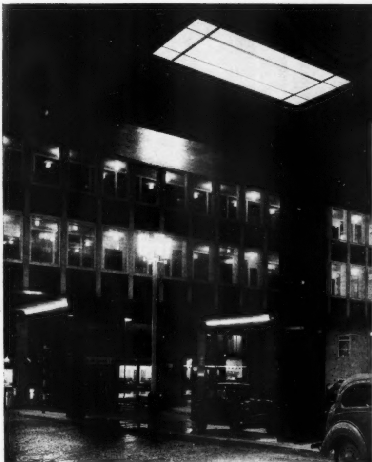
Bowater House, Knightsbridge. Architects: Guy Morgan and Partners. 8' x 4' recessed lighting fittings over public road. Centre panel of each is close reeded 'Perspex' 3/16" thick. Surrounding panels are .040 'Perspex'. Each fitting holds two 5' 80 watt fluorescent lamps. The lay-lights are hinged for maintenance — 'Perspex' being light enough to allow this. Set of amenity Lighting Columns with .040 'Perspex' diffusers and continuous fittings with .040 'Perspex' diffusers and black 'Perspex' ends under the low block in background. All fittings by Troughton and Young (Lighting) Ltd., Knightsbridge, London.
