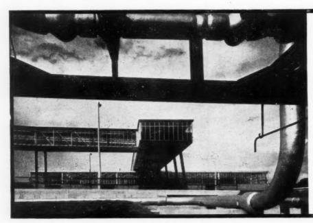
The new Heinz factory at Wigan is the largest factory to be built in Britain since the war. Shown here is the ancillary can factory, clad in Williams & Williams are Williams are gear-opening lights are gear-operated to give critical control of ventilation.
