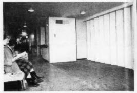
Viewpoint 15: sliding-folding doors into the casualty department allow ambulances to back up under cover right into the building. This is one of the few key points where the floor slab heating is supplemented, in this case by warm air batteries.
