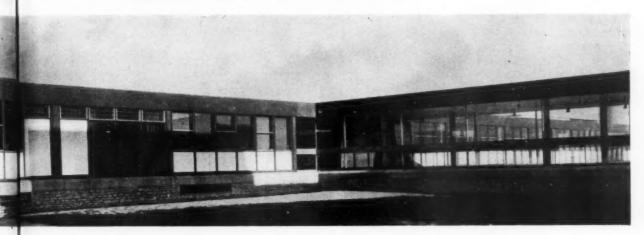
Viewpoint 3: the ophthalmic clinic from the east: external facings have been chosen for low maintenance, the concrete frame being finished with slate slabs, with bronze mullions, between. Windows are vertically sliding aluminium sashes, adjustable glass lowers and fixed double glazing. Solid panels below the sills are in white opaque glass throughout, with plastic-faced plywood inner skin and aluminium foil-backed wood-wool slabs between, for thermal insulation.
