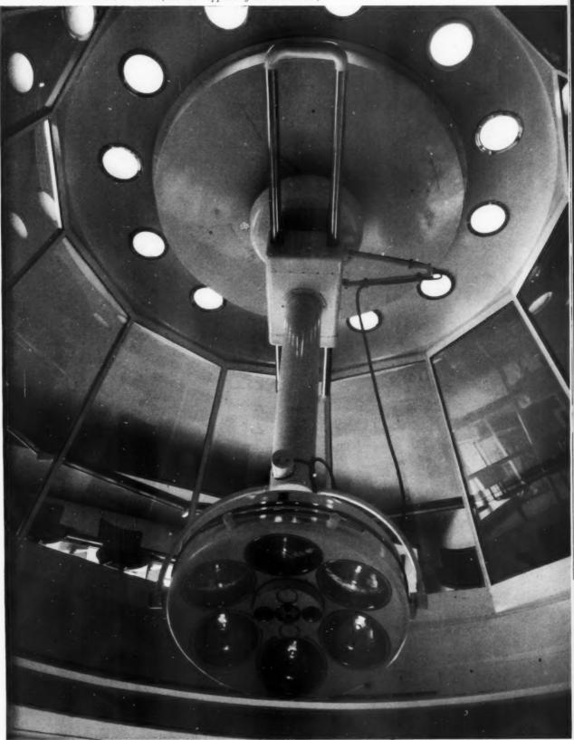
The chief interest of this detail is in the slim glazing members which also support the timber elbow rest, and the economical detailing of the kerb on which the glazing rests.
