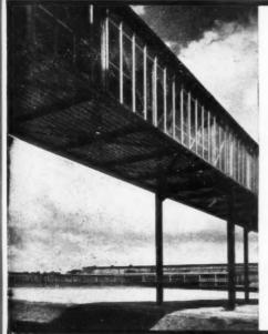
WILLIAMS & WILLIAMS ALUMINEX SIDEWALL GLAZING HAS BEEN USED TO CLAD
