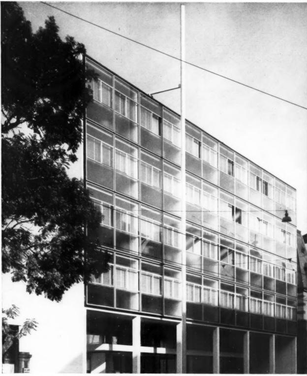
This is an interesting essay into the decorative possibilities of fluorescent light tubes, which in this case are housed in an aluminium mast fabricated and erected in one piece.
