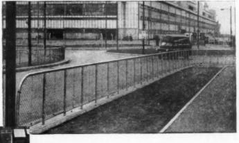
Above: Nearly a mile of specially designed guardrailing was supplied and erected by us for the approach road to the Ford Motor Co's new foundry at Dagenham. Infilled with 2-inch woven diamond mesh. Contractors: John Laing & Sons Ltd.
