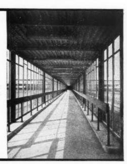
and is linked to it by a service gantry which feeds the finished cans into the appropriate stage of production process.
