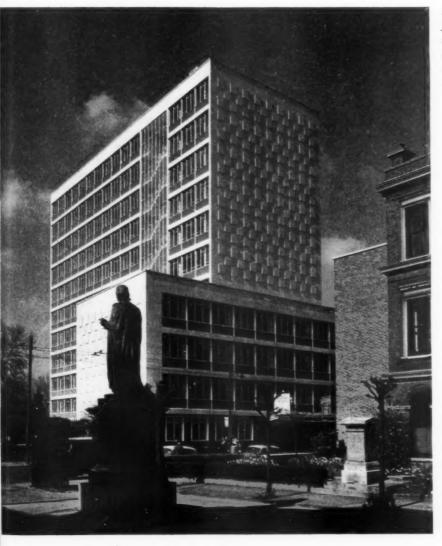
Besides the glazing, four different facing materials can be seen in this view: artificial stone, exposed aggregate (spandrels of tall block), vitreous mosaic (spandrels of low block) and polished marble (ground floor of low block).
