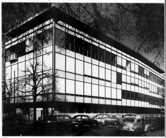
Even in this country it is probably necessary to provide some form of sun control on west-facing facades which have large areas of glass. The most effective form of sun control is a movable sun-breaker fixed outside the glass. In this example (which is typical of current Continental practice) sun control is provided by an external roller blind which is guided by the mullions. Architects' Journal 3.3.60
