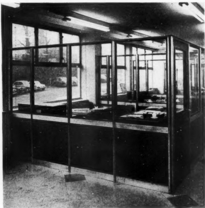
Above and below: purpose-made movable partitions designed by the architects.
