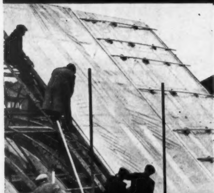
Scaffold boards 3' 10 1/2" apart were lashed diagonally to purlins at 5' centres. 'Visqueen' was unreeled over the boards and battened down with 1 1/2" x 1/2" slate laths.
