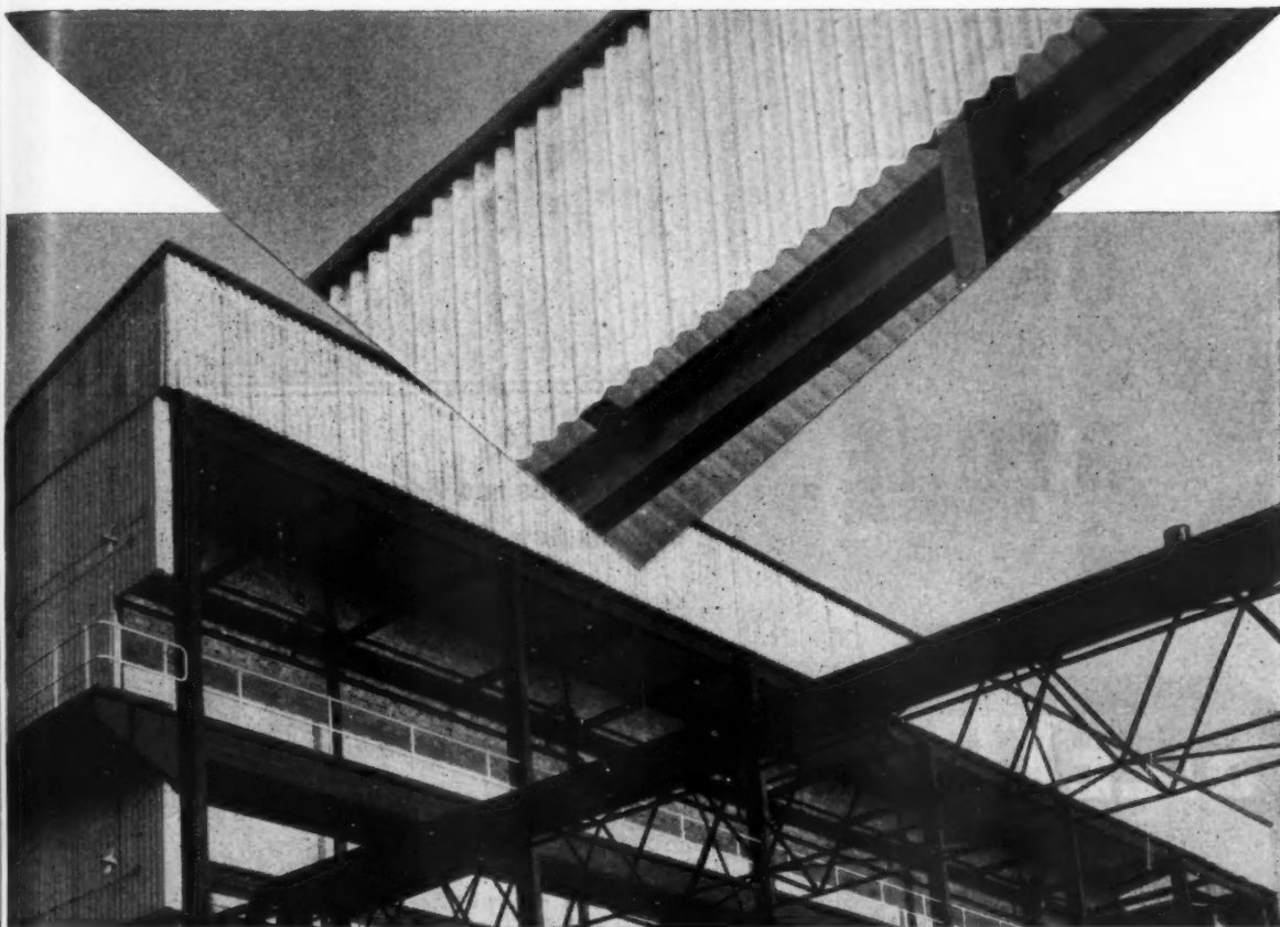
FILON cladding protects the machinery bays of a new factory on the East coast.
