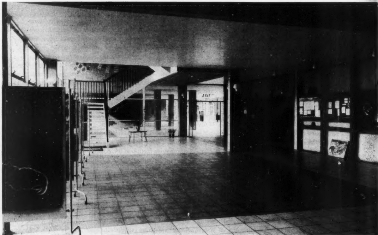
Panels next to the classroom doors are of plastered 2½-in. concrete block, and obvious movement between the door frame and the panel has resulted in cracking in a good many cases. The melamine plastic-faced doors, however, show no sign of wear and look extremely well, as does the hardwood framing.
