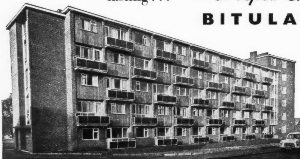
The Wilbert Lane Flats at Beverley, with Keruing cladding treated with Transparent Bitulacum 3502 Satin Finish. Photograph by permission of Messrs. Anthony Steel and Owen A.A.R.I.B.A.
