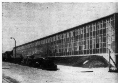
I.C.T. factory at Castlereagh with aluminium curtain walling construction. One extruded section was used to frame the curtain wall at head, sill and jambs. Architects: Smyth & Cowser, R.F.R.I.B.A.
