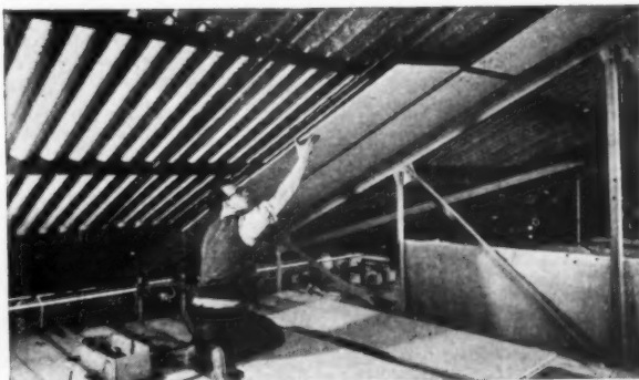
Erection by Specialist Contractors, Messrs. Sundeala Board Co. Ltd. Architects: Messrs. Farmer & Dark of Tufton St., S.W.1
