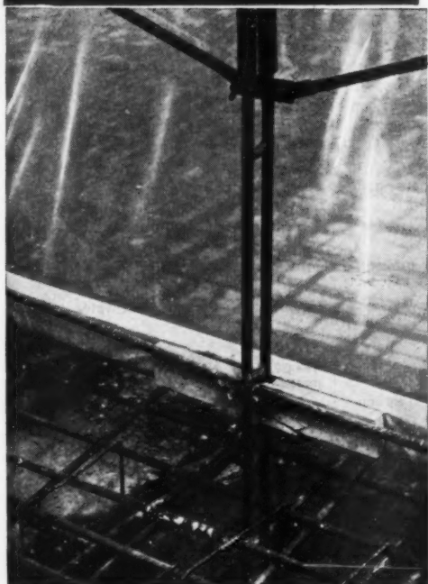
Method of fixing the sheeting to the framework. The 'Visqueen' was wrapped round rough-sawn timber battens and nailed at intervals. These were then fastened to wood blocks already secured to the metal work.
