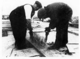
Fig. 9. Nails being pneumatically driven home into one of the portal frames on site before erection.
