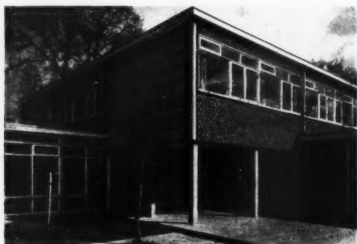
"with Notts schools stanchions are deliberately hidden behind the windows and a variety of claddings."
