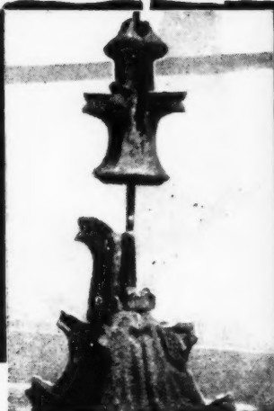
Cap of pinions at Houses of Parliament and by corrosion of iron central rod (after welds replaced by "Delta" Bronze No. IV)
