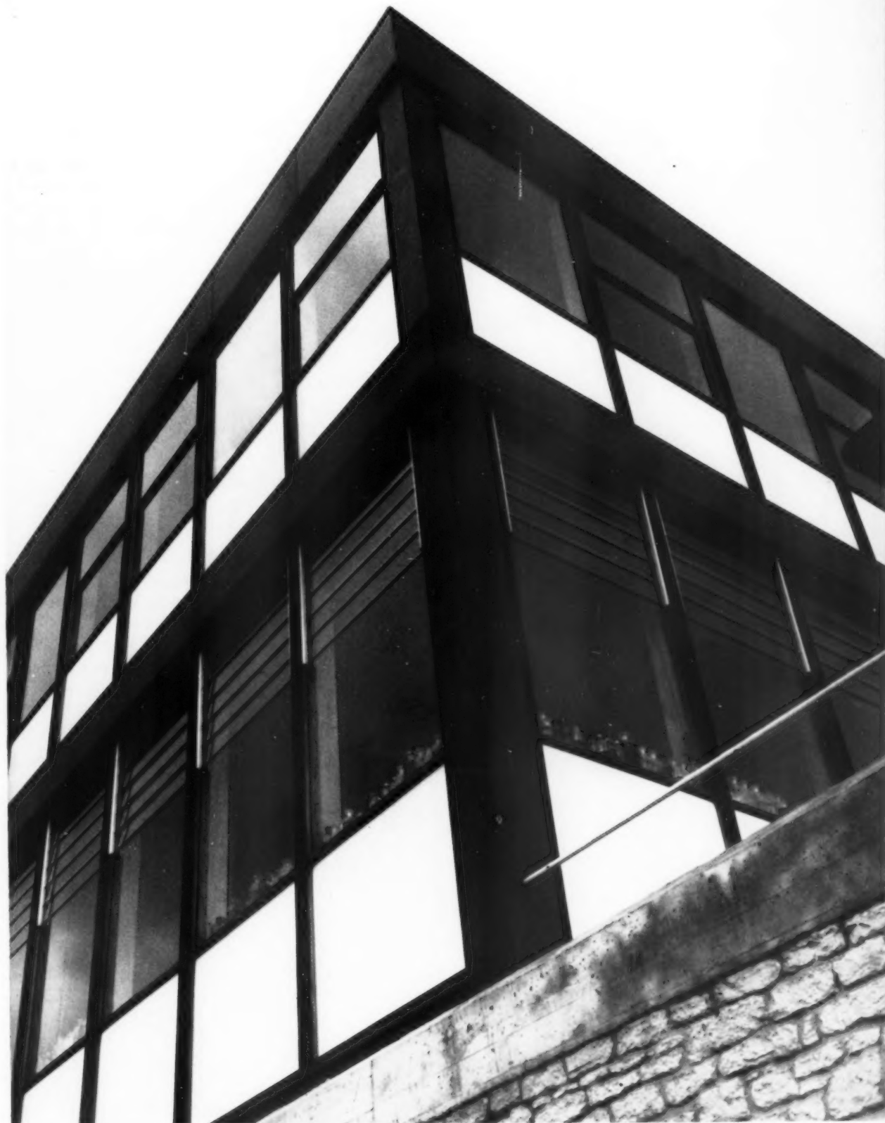
This detail is concerned with the slate fascias and column cladding and the attendant flashings. Note the recession of the slate to receive the flashing, a refinement made necessary by the smoothness and precision of the slate. The facing to the horizontal string at first floor level (Section B-B) is restrained by cramps similar to those used on the fascia (section C-C).
