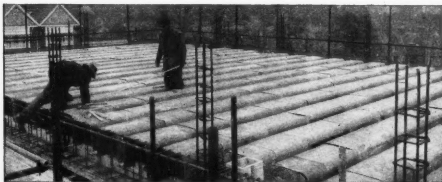
Hollow steel mould being placed in position
