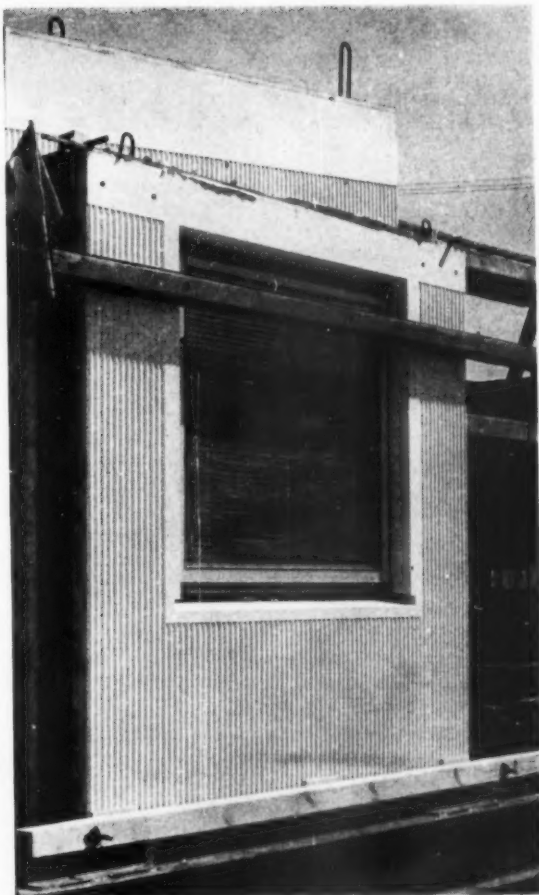
Fig. 2. External wall unit for a Larsen & Nielsen project. The surface finishes are of high quality.
