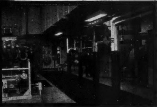
Full cooling and full heating may be demanded simultaneously by different zones of this complex air conditioning plant.
