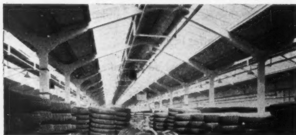
Croft Precast Reinforced Portal Concrete Frames for Industrial Buildings are quick and easy to erect with great permanent strength.
