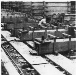
Precast units under manufacture at Messrs. W. & C. French's factory awaiting delivery to the site.
