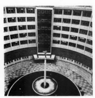
The central garden, below which is the tele-recording studio. The steel-framed structure is faced with mosaic and the brick spandrels with pale grey faience. The studio control area is expressed externally as a storey-high band of pale green mosaic, with a lined pattern in scarlet. The south hall staircase, behind which is the "central wedge" is also faced with mosaic. The floor of the garden is paved to allow easy access for fire fighting.
