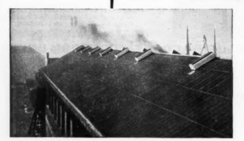
Exhaust gases from fork lift trucks and lorries were once a major problem in this storage shed. Colt experts were called in to make a scientific analysis and on their recommendation a series of Colt S.R.C./3080 High Duty Extract Ventilators was installed. Fumes no longer bother anyone.
