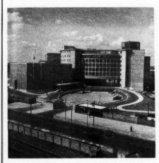
View from Main Entrance: Studio I on left with covered way for studio audiences; section of inner "drum" of office, centre. A "spur" extension will be connected to the existing building on the right.
