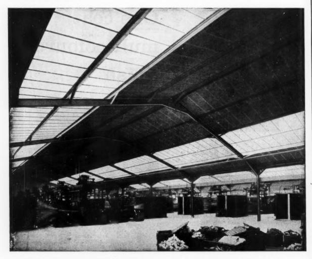
This is a typical Clearspan steel portal roof—light, clear and spacious. Yet Clearspan costs less than other forms of construction. As the subject of careful cost comparison in the "Architects' Journal", June 5th, Clearspan showed a saving of 3s. 4d. per square foot over its nearest rival, a total saving of £7,000.
