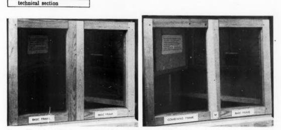
Fig. 7. Two-light window frames constructed from two basic frames (left) and from combining frames (right).
