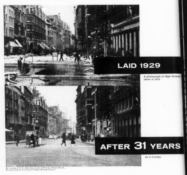
Laid in the spring of 1929, this section of High Holborn, London, is of concrete construction reinforced with BRC Fabric. Although this road has had to take its full share of the terrific increase in London's traffic, the only maintenance has been the laying of an asphalt carpet on top of the reinforced concrete. It is as capable of bearing the heavy loads of today as when it was first laid more than 31 years ago.
