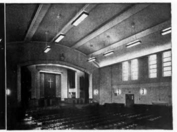
Lighting units, each weighing over 2 cwt., are serviced by means of L.E.F. Raising & Lowering Gear at the Leysian Mission Hall.
