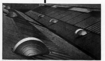
The pressing of rubber mouldings at the large factory of the John Bull Rubber Co. Ltd. was causing condensation under certain climatic conditions and sections of the structure and floor were covered with moisture. This raised humidity and created unpleasant working conditions. Colt were called in and after a survey recommended the installation of Inflow Units and SRC 2046 ventilators.
