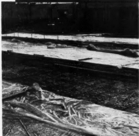
The 'Visqueen' sheet is shown being used to lay the ground floor slab of the new Preston Road factory at Stevenage. Although 10 ft. by 16 ft. 'Visqueen' was used on this site, 7 ft. by 10 ft. sheets are available. F.R.I.E.A. & Partners, Consultants, Stevenage, Herts. (South Essex) Ltd.
