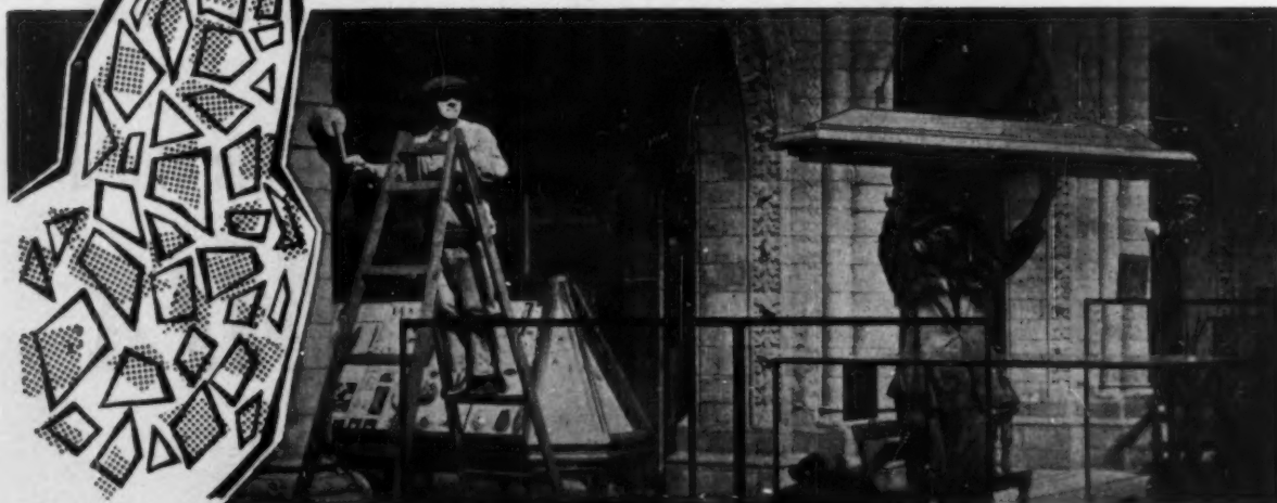
Lights being serviced at the Natural History Museum by means of L.E.F. Raising and Lowering Gear.
