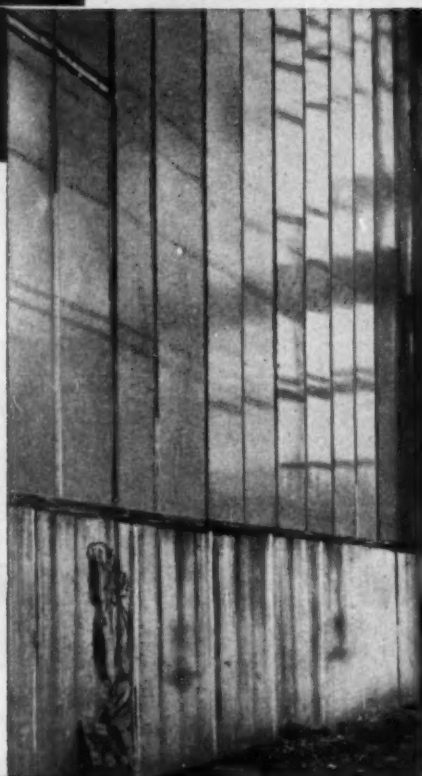
The foundry at Midland Rollmakers Ltd., Crewe, protected from the weather by a screen of 'Visqueen' building sheet after the demolition of a complete wall to make way for extensions. The sheeting is supported on vertical timbers clipped to the scaffolding. Contractor: Sir Alfred McAlpine & Son Ltd. Consulting Engineers: Sir Alexander Gibb & Partners.
