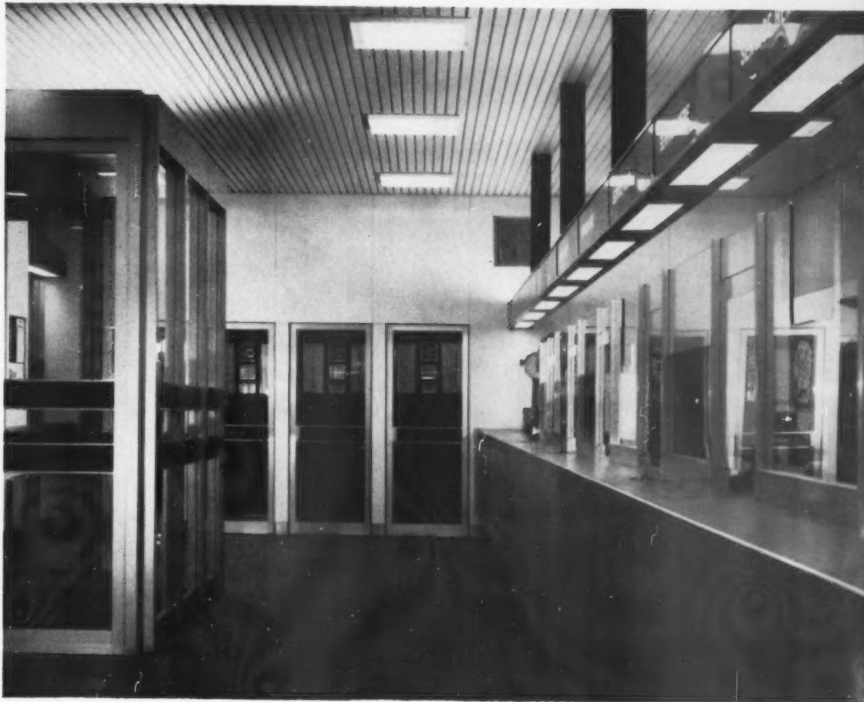
The fluorescent tubes illuminate the counter positions, through plastic louvers, and the signs above them.
