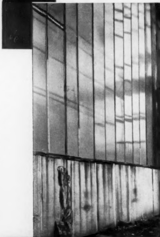
The foundry at Midland Rollmakers Ltd., Crewe, protected from the weather by a screen of 'Visqueen' building sheet after the demolition of a complete wall to make way for extensions. The sheeting is supported on vertical timbers clipped to the scaffolding. Contractor: Sir Alfred McAlpine & Son Ltd. Consulting Engineers: Sir Alexander Gibb & Partners.
