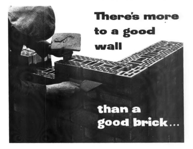
and that means the mortar - for the strength, stability and watertightness of the wall depends on the type of mortar used. In the soft state, the mortar must be highly plastic so that it spreads with ease and allows the bricks to be cushioned easily into position. It should hold together well and it must also have good water retentivity to prevent the bricks sucking the water out of the mortar too quickly so that the mortar does not stiffen before the bricks are thoroughly bedded and bonded.
