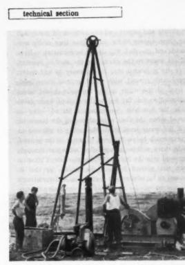
Fig. 1. Typical portable boring rig suitable for most site investigation
