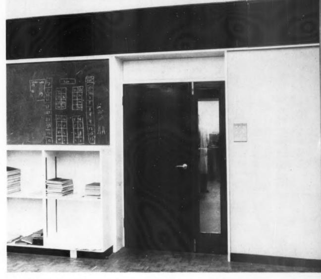
It is now becoming common practice to use a normal width door in conjunction with a narrow glazed panel. This useful variation shows the vision panel treated as a separate leaf which is secured during normal use by substantial flush lever bolts top and bottom, but which can be opened on the rare occasion when something bulky has to be brought through. (32) DOORS: 47 is expendable, and has a limited period fixed prices, price rings and monopolies
