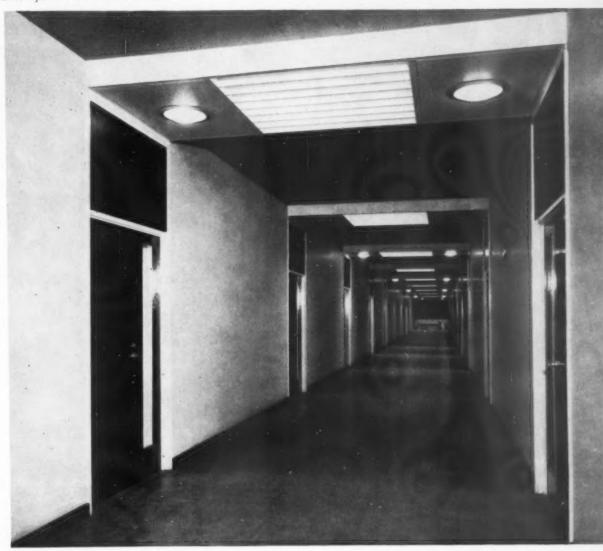
This detail shows a sensible way of combining natural and artificial light in a long corridor. Note the alignment of the lighting unit with doorways and the use of transverse ceiling elements to reduce the apparent length and increase the apparent width of the corridor. (37) LIGHTING: 24
