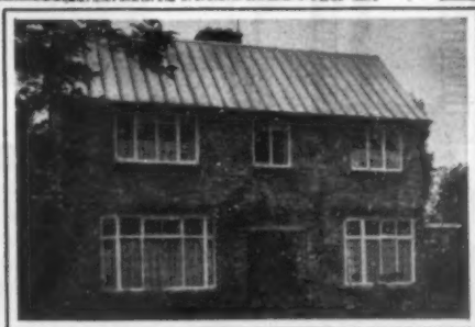
'Economy' copper roofing on the house of J. Holdsworth Esq., Aylestone, Leicester.
