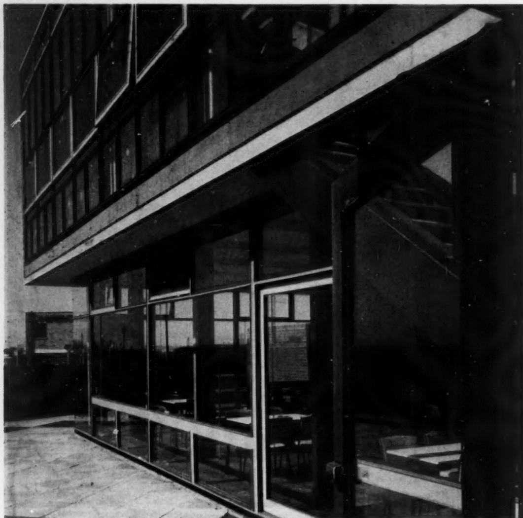
The glazed wall to the staff room returns with a shop-front detail of glass to glass. This is the only place where two glazed walls meet on an external angle. The great variety of details, frequently doing similar jobs, is slightly disconcerting in so small a building
