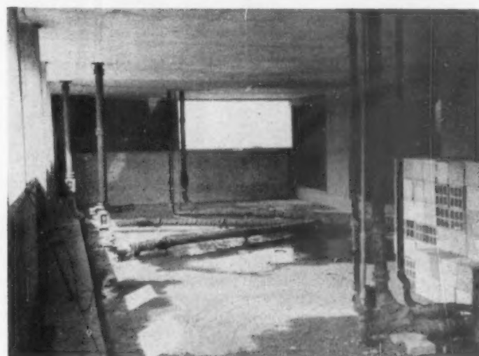
Fig. 6. Drainage pipes brought across the deep first-floor tray so as to avoid down-pipes at perimeter of open ground floor
